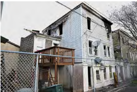
Rehabilitation and demo of residential homes in Ducktown
