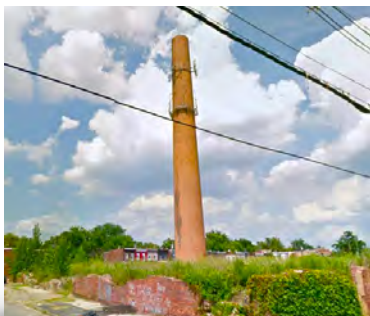
Site of former Croft Mills factory, corner of Broadway & Jefferson
