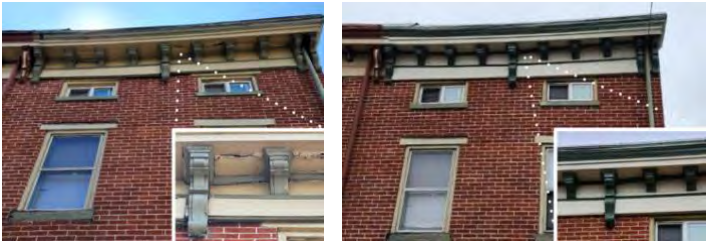
North Stockton Street cornice repair – before & after
