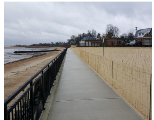
Old Bridge MUA Laurence Harbor Bulkhead and Walkway
