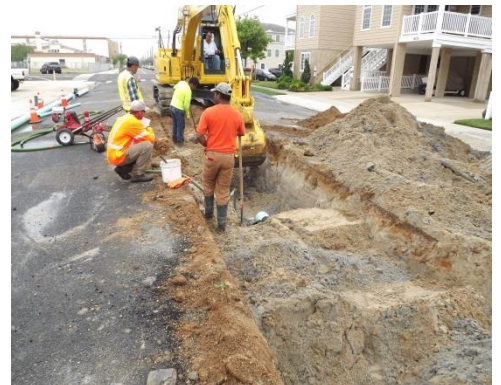
North Wildwood Sewer, Storm and Street Restoration
