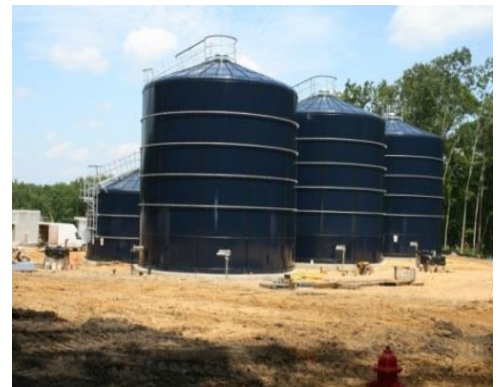
Construction of Storage Tanks at the Jackson Twp. MUA
