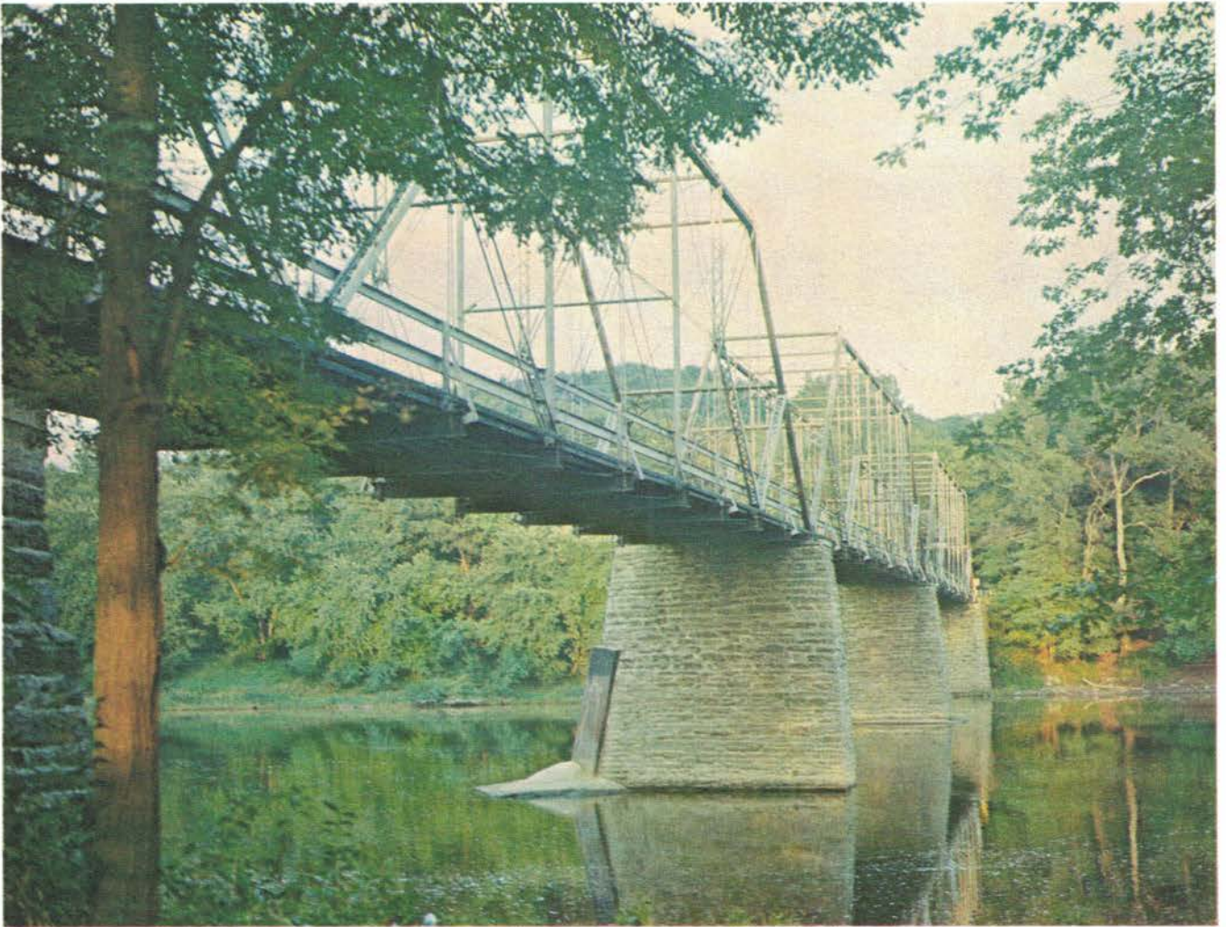
The toll bridge crossing Delaware at Dingman's Ferry, from Pennsylvania side. Area would be inundated by Tocks Island reservoir.
