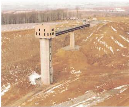
Water spews from the base of Merrill Creek's inlet/outlet tower as filling of the 15 billion-gallon reservoir began in March of 1988.
