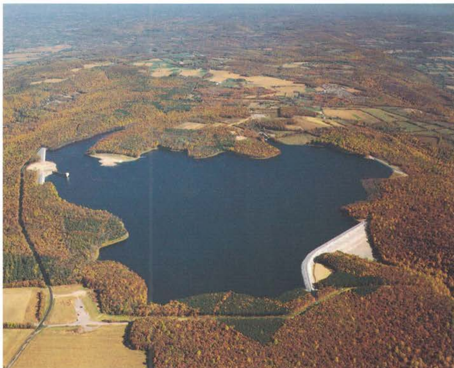
Merrill Creek Reservoir, another by-product of the “Good Faith” agreement, was completed in late 1987, then filled with water pumped from the Delaware River. The 650-acre impoundment is designed to release water back into the Delaware during low flow periods to compensate for depletive water use at electric generating plants owned by seven utilities.
