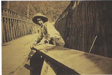
The water trunk was removed in 1930 and replaced with a wood deck. A worker pauses during the conversion project. (Photo by Haupt)
