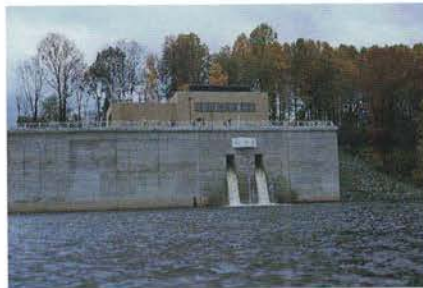
Water flows from the Merrill Creek pumphouse into the Delaware River during a test release in October of 1988.
