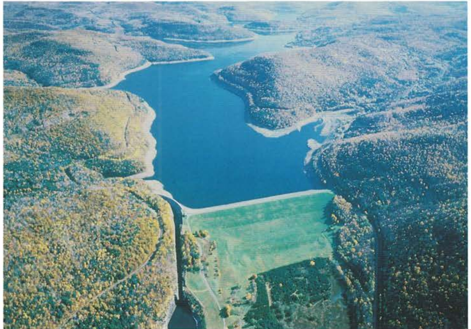
Releases are made from water supply reservoirs during low flow conditions in basin rivers to prevent salty water from migrating upstream from the Delaware Bay and contaminating aquifers in southern New Jersey. Releases also are made to improve water quality and protect basin fisheries by lowering in-stream temperatures and increasing dissolved oxygen levels. Shown above is the Pepacton Reservoir, a 140 billion-gallon impoundment located on the Delaware's East Branch and owned and operated by New York City. (Photo courtesy of John Goerg, NYDEC)
