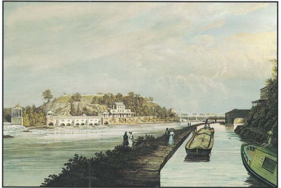
George Lehman's 1842 watercolor depicts the eight arched openings through which the water exited the Water Works after driving the water wheels, and later the turbines. Note the stairs leading up to the reservoir atop "Faire Mount." To the right is the canal built by the City of Philadelphia for the Schuylkill Navigation Co. (Courtesy, CIGNA Museum and Art Collection)
