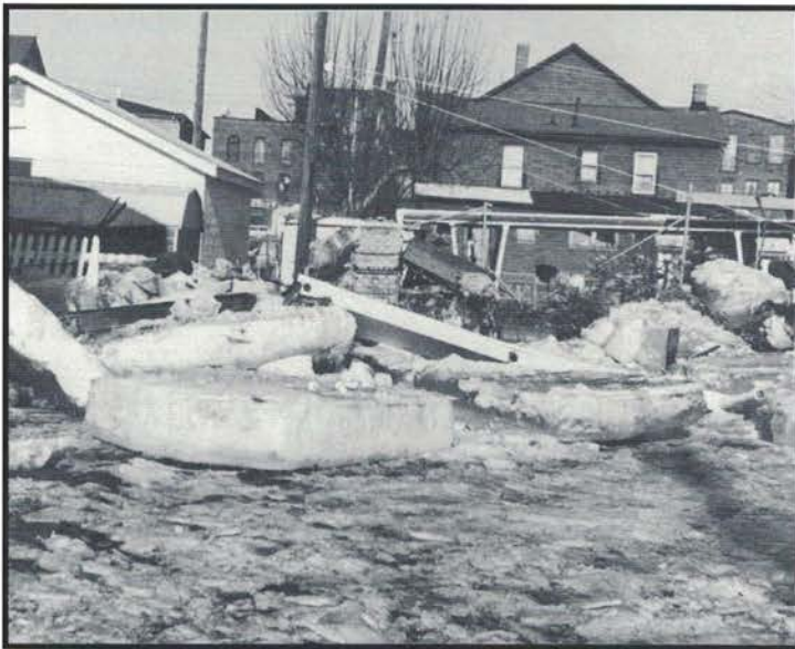
Rapidly rising waters heaved huge slabs of ice into Port Jervis during the 1981 flood. The ice punched through cinderblock and brick walls destroying or seriously damaging many structures. (Courtesy of the Minisink Valley Historical Society, Port Jervis, N.Y.; photos by R.G. Tarbell)
