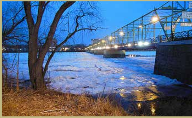
Ice jam on the Delaware River at the Calhoun Street Bridge in January 2014. This is a view from Morrisville, Pa. looking across the river towards Trenton, N.J. Additional information about the ice jam can be found in the Annual Hydrologic Conditions Summary beginning on page 12.
