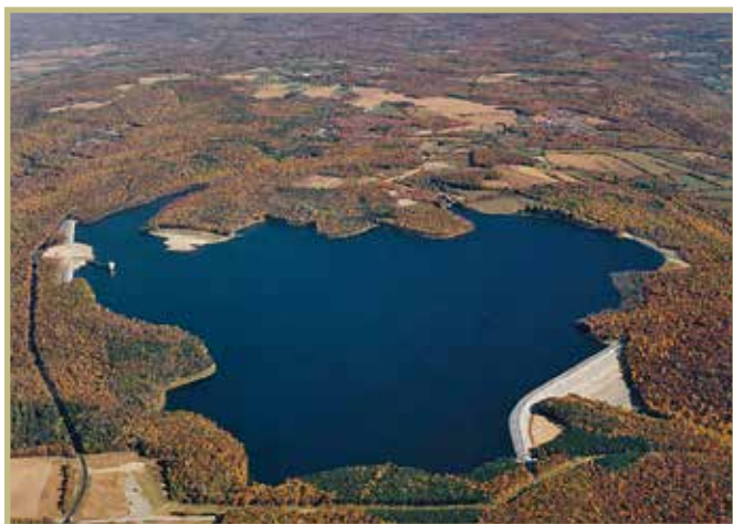
The Merrill Creek Reservoir was designed to provide makeup water for riverbank electric generating plants during low flow conditions on the Delaware. It became operational in 1988.
