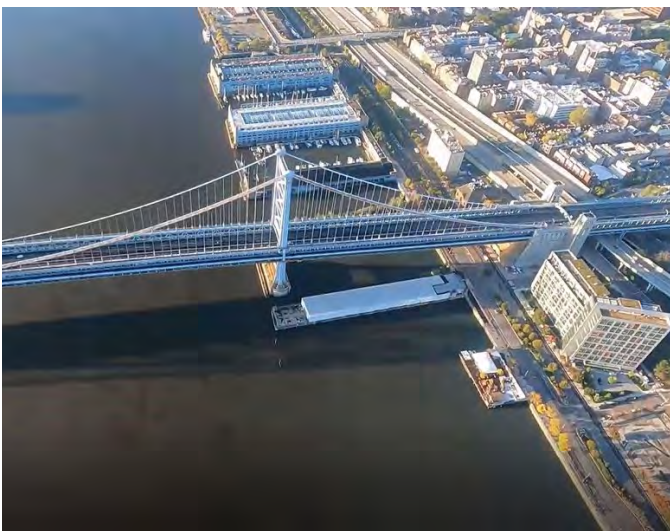
Ben Franklin Bridge going into Philadelphia, Pa.
