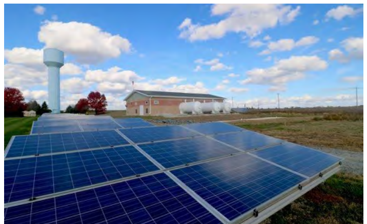
Artesian Water's Hyetts Corner Water Treatment Plant in Southern New Castle County, Del. Courtesy of Artesian Water.
