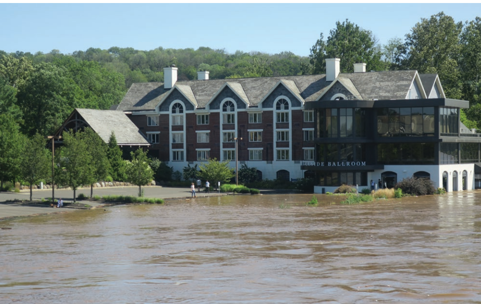
Ida flooding, September 2021
