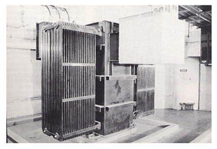
Figure 1 Liquid-filled Transformer Pad-mounted may contain askarel
