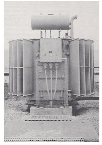
Figure 3 Liquid-filled Transformer with Conservator Tank
