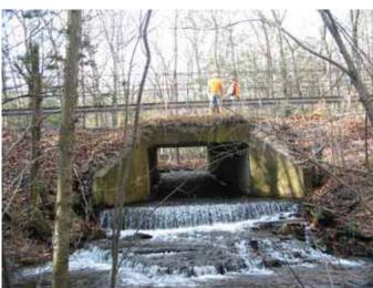
Figure 9 - Cranberry Creek at Route 191 crossing. This location receives a large quantity of road runoff, which should be managed to reduce introduction of pollutants to stream.
