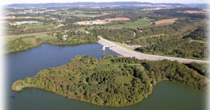
Photo courtesy of the U.S. Army Corps of Engineers
