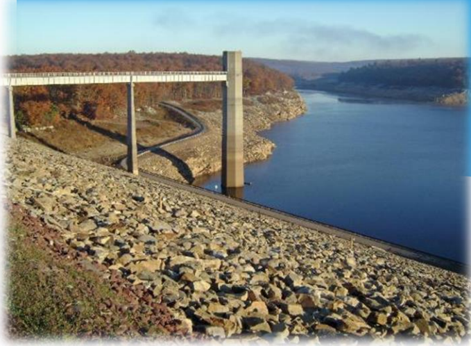
Frances E. Walter Reservoir, USACE Luzerne County, PA Photo courtesy of the U.S. Army Corps of Engineers
