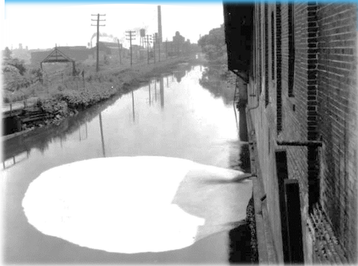
Slaughterhouses discharging in 1928 (courtesy of the Phila. Water Dept. Historic Collection)
