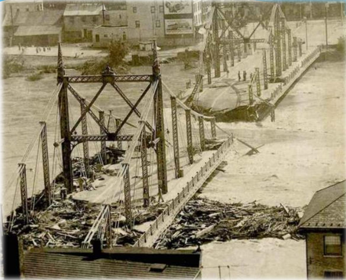
Easton-Phillipsburg free bridge in 1955 (file photo courtesy of lehighvalleylive.com)
