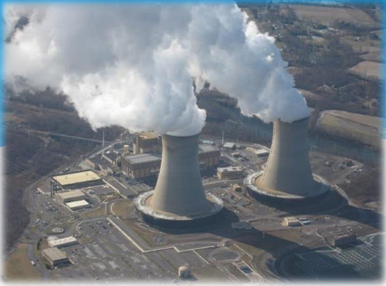
Exelon Limerick Generating Station, Montgomery County, Pa.
