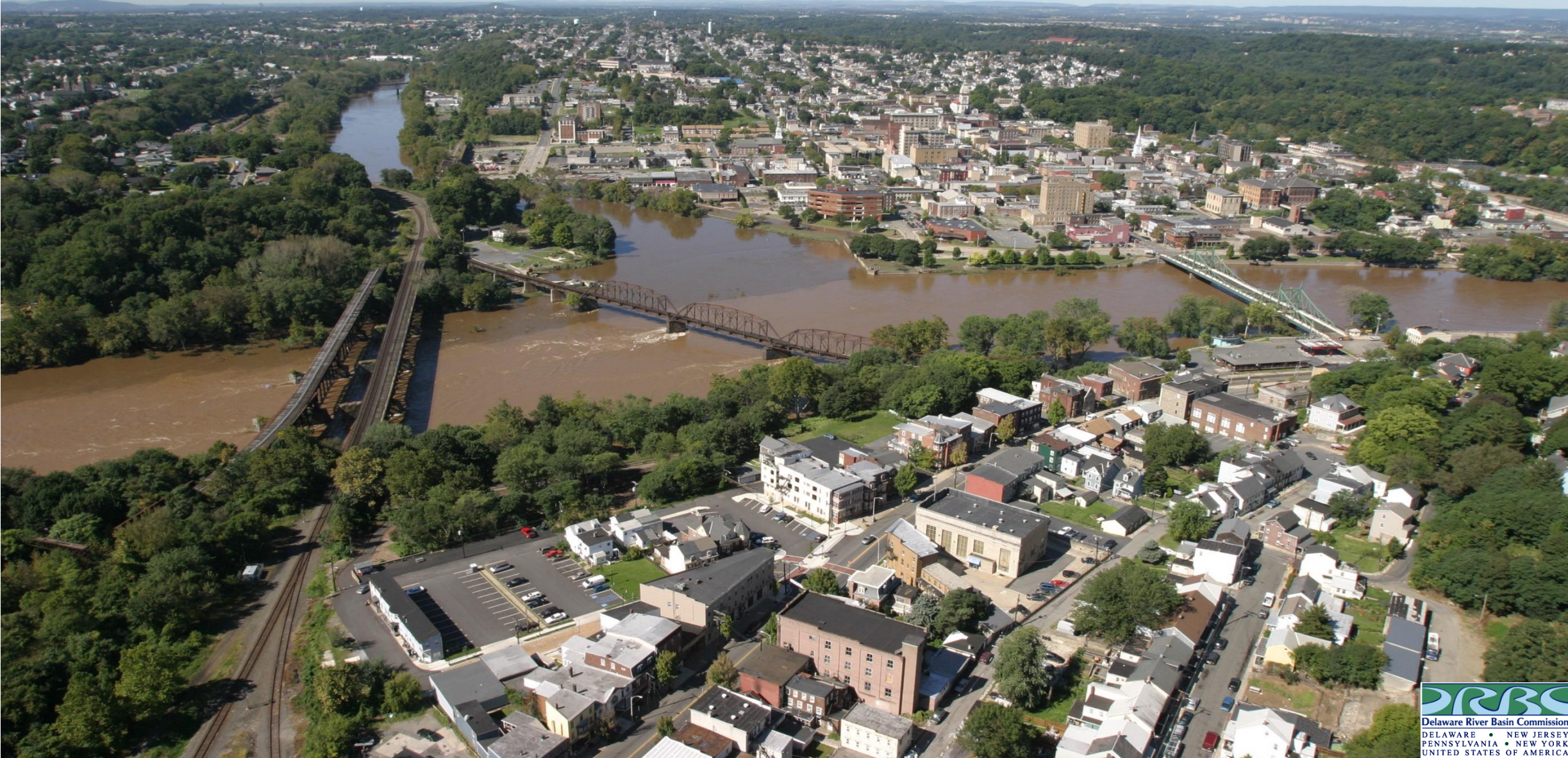
Photo: U.S. Army Corps of Engineers Sept. 2004 Flood, Easton-Phillipsburg
