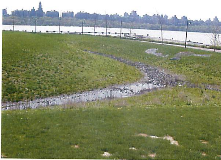
Photograph 1: Retention basin at the former landfill
