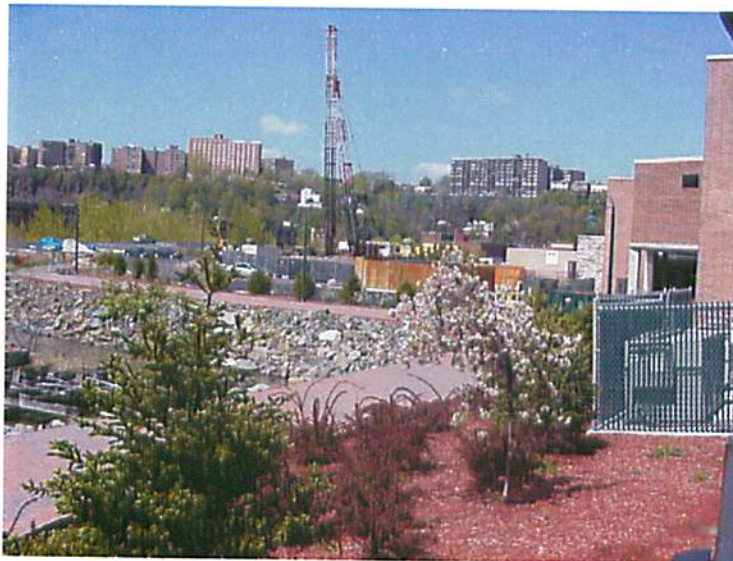
Photograph 2: Construction of Building 7
