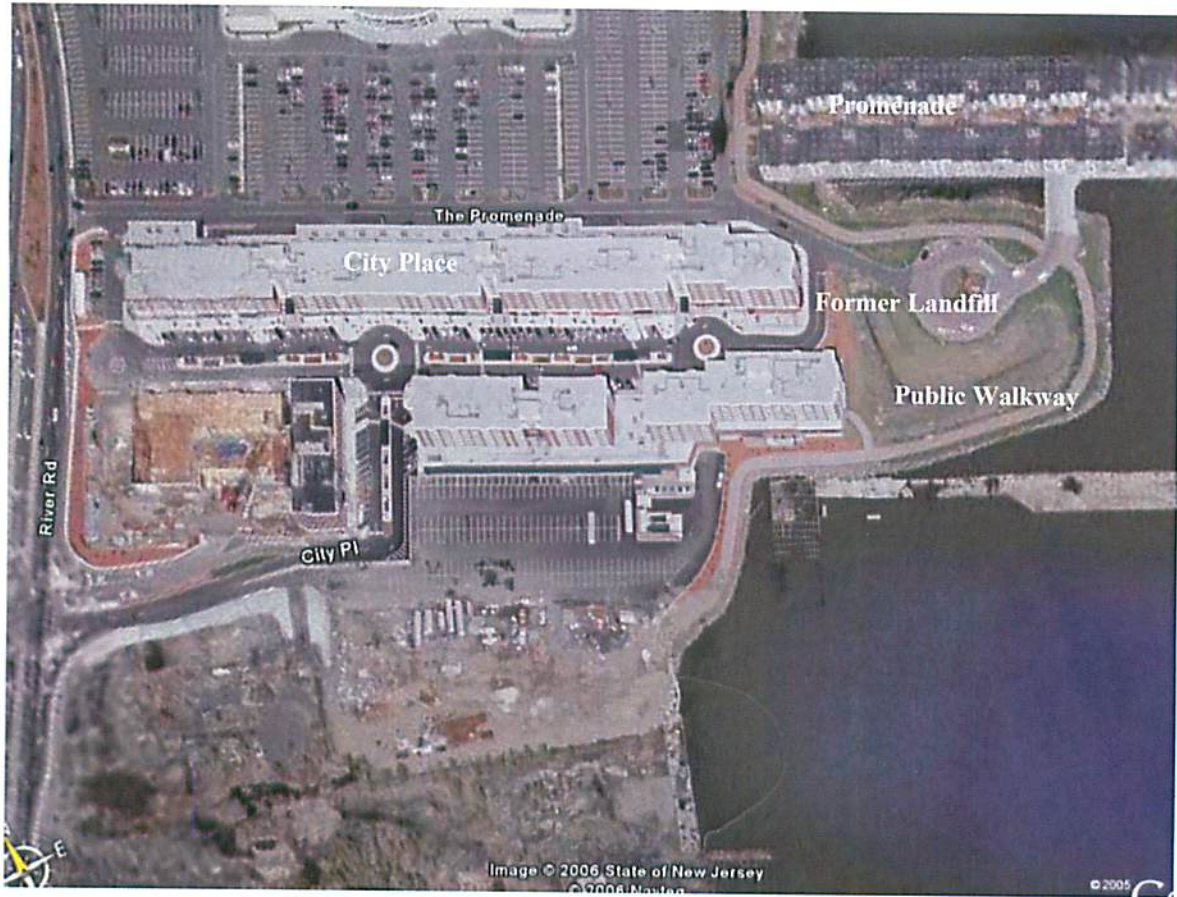
Figure 2: Location of the Promenade in relation to the former landfill
