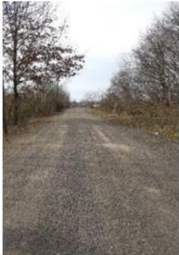
Access Road between Main building and Grand Sprute Run
