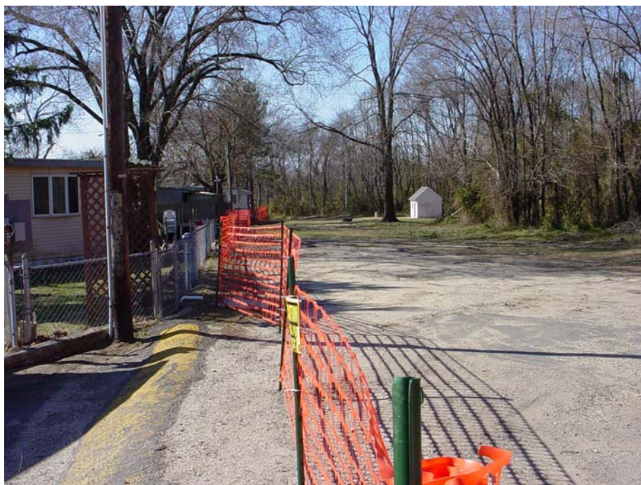
Photograph 9: Temporary fencing restricting access to the open area present behind the homes in the Willow Woods MHC
