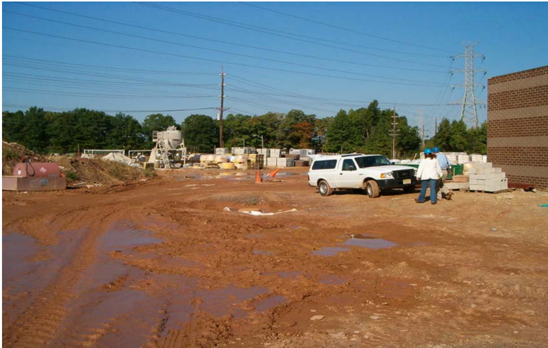
Photograph 2: View of construction area on northwest side of NBTHS.
