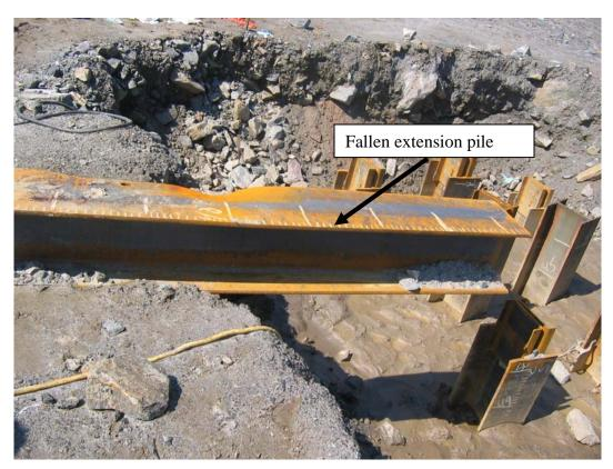
Figure 3: Fallen extension pile.
