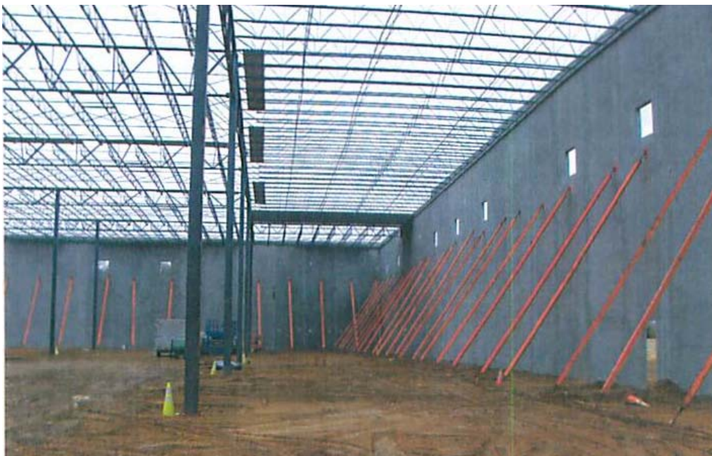
FIGURE 1. Incident site; inside and outside views of construction site.
