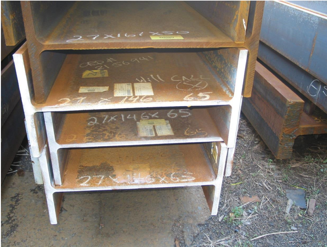
FIGURE 5. Stable, centered stack of steel beams.
