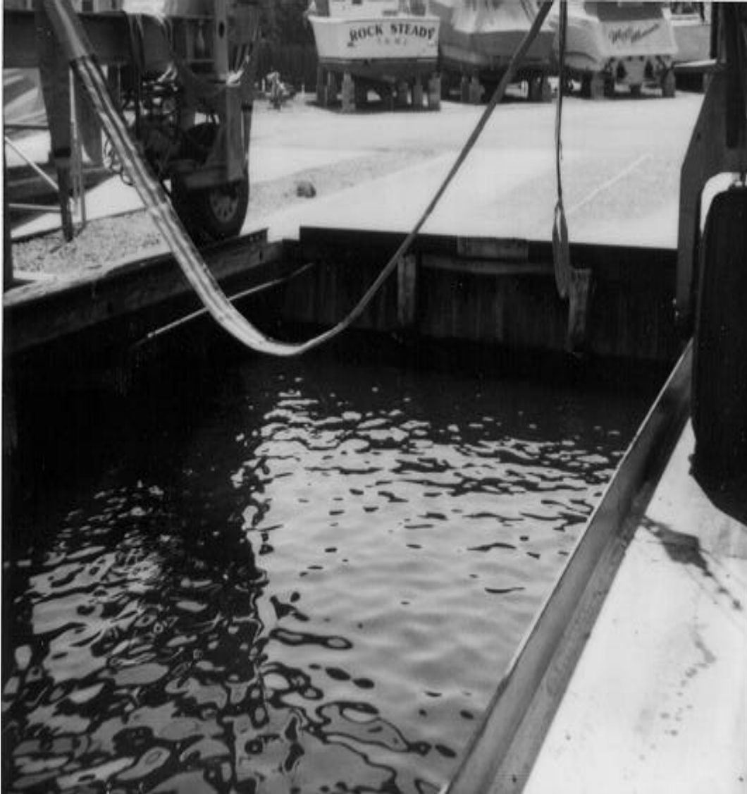
Photograph #1 View of Travel Lift Dock Area
