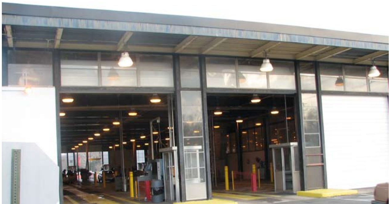
Bakers Basin Inspection Facility in Lawrence Township
