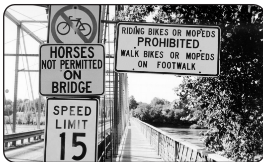
Obey the posted regulations on bridges.
