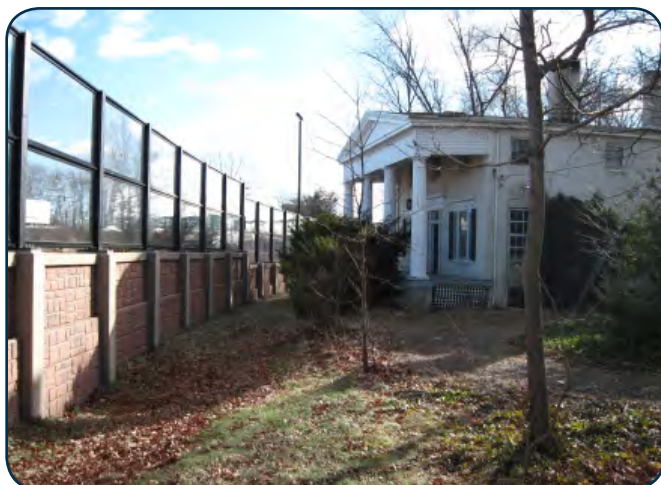
Clear noise wall panels at the Agnew House, Route 18, New Brunswick, Middlesex County. (Courtesy of NJDOT.)
