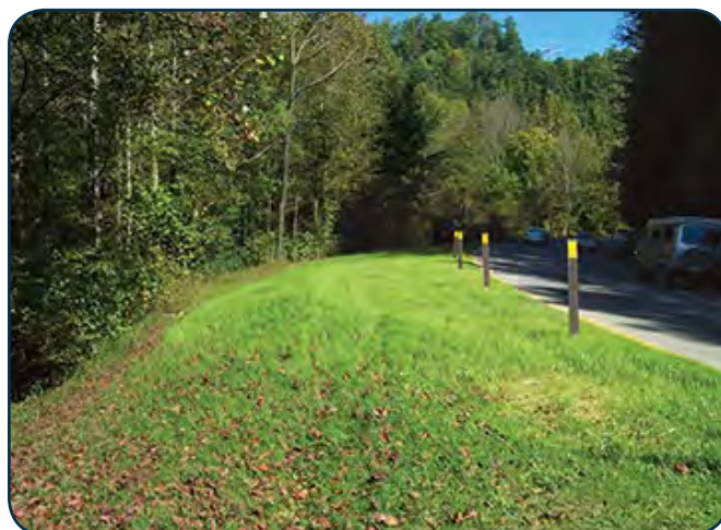
Construction of a stabilized grass pulloff area, with a geoblock base, along the Foothills Parkway in Great Smoky Mountains State Park, Tennessee, during (left) and after construction (right). (Courtesy of the Federal Highway Administration.)
