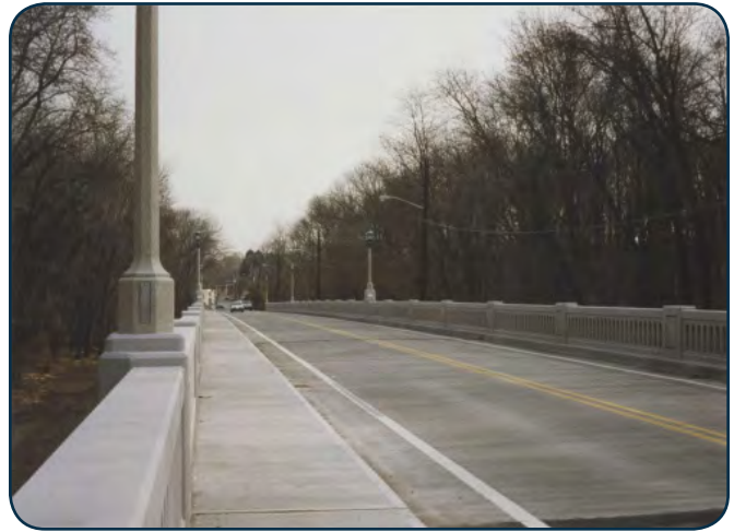
Millstone Causeway after rehabilitation. The perforated parapet with scored piers reflects the design of the historic bridge. (Courtesy of NJHPO).
