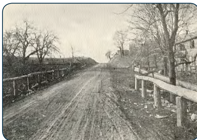
Morris Turnpike, Lopatcong Township, Warren County, after improvements, date unknown. (Courtesy of NJDOT.)
