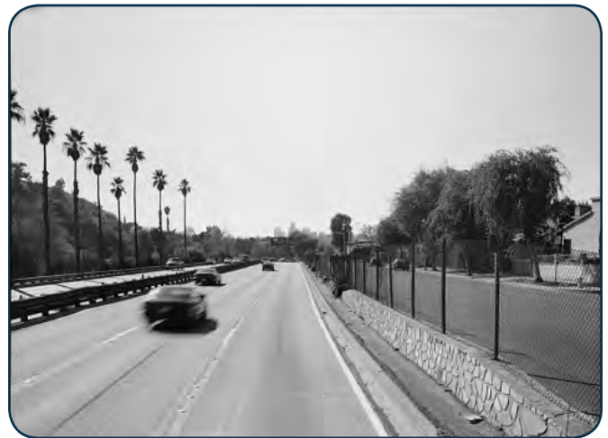
Arroyo Seco Parkway at Avenue 26. Note the stone guide rail with chainlink fence (HAER CA-265. National Park Service).
