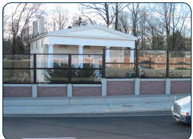
Clear noise wall panels at the Agnew House, Route 18, New Brunswick, Middlesex County. (Courtesy of NJDOT.)
