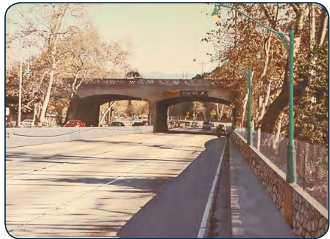
Mock-up of proposed improvements, including stone side barriers and lighting inspired by historic fixtures. (Courtesy of Cal Trans.)
