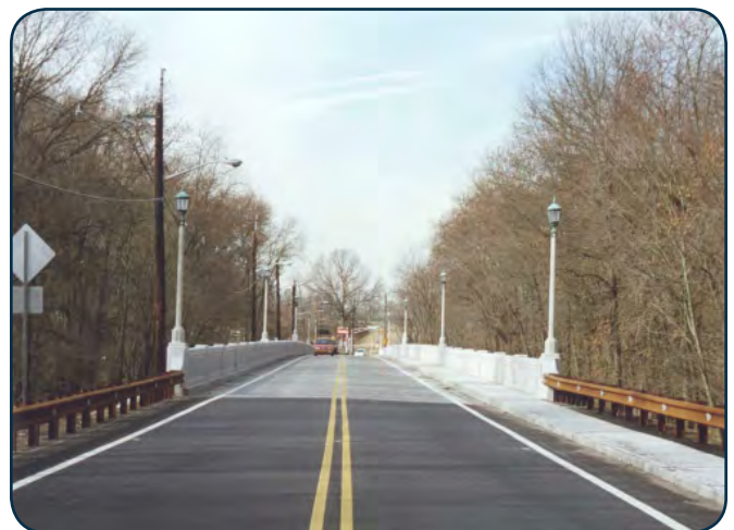
Millstone Causeway after rehabilitaion. Guide rails are brown to blend with surrounding trees, and light fixtures are modeled after those on the bridge prior to renovation. (Courtesy of NJHPO).
