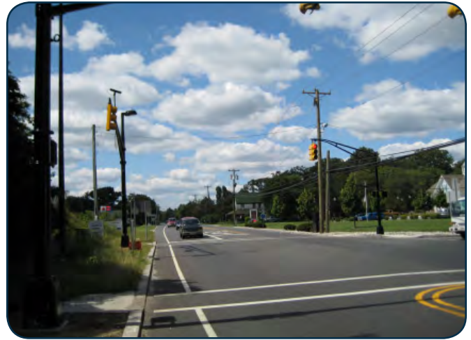
Left turn lanes were accommodated within the existing roadway by incorporating existing shoulder areas. (Courtesy of NJDOT).
