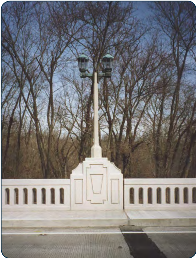
This replacement light fixture on Millstone Causeway in Millstone, Somerset County, was modeled after the original fixtures that remained on the bridge prior to the replacement of the superstructure. (Courtesy of NJDOT.)
