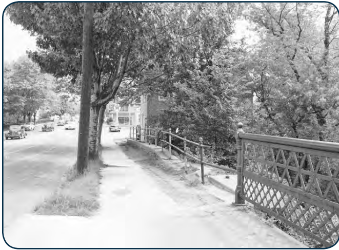
Route 45 bridge over Woodbury Creek, Woodbury, Gloucester County, 1954. (Courtesy of NJDOT.)
