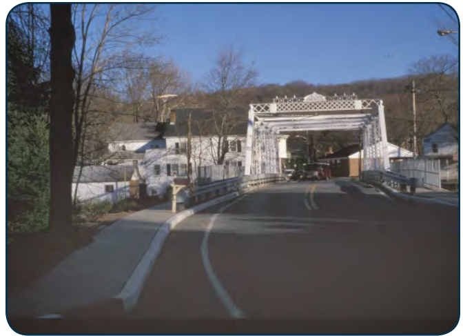
The rehabilitated and widened Califon Bridge, c. 1986. (Courtesy of NJHPO).
