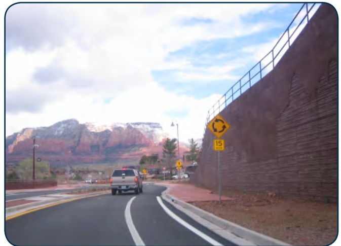
The formliner design for this retaining wall reflects the “red rocks” of Sedona, Arizona. Similar technology can be used to implement appropriate interpretation on noise walls. (Courtesy of KSK.)
