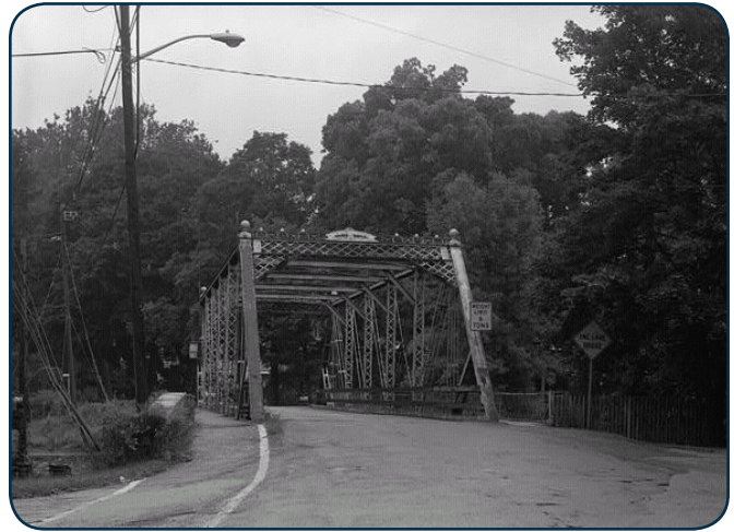
HAER documentation. Califon bridge before rehabilitation. (Courtesy of NJHPO).
