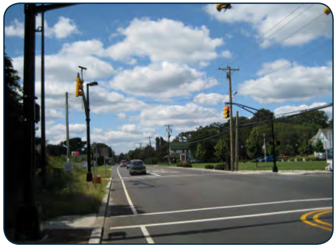
Black powder coated mast lighting and utility cabinets (right of center, next to the telephone pole) with landscaping can minimize visual intrusions in historic areas. This is Route 47 in Dennisville, Cape May County. (Courtesy of NJDOT.)
