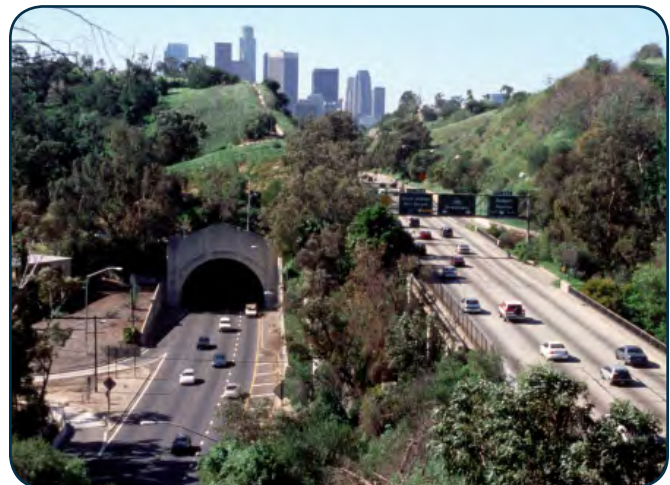
Arroyo Seco Parkway (left) through Elysian Park. (Courtesy of Cal Trans.)
