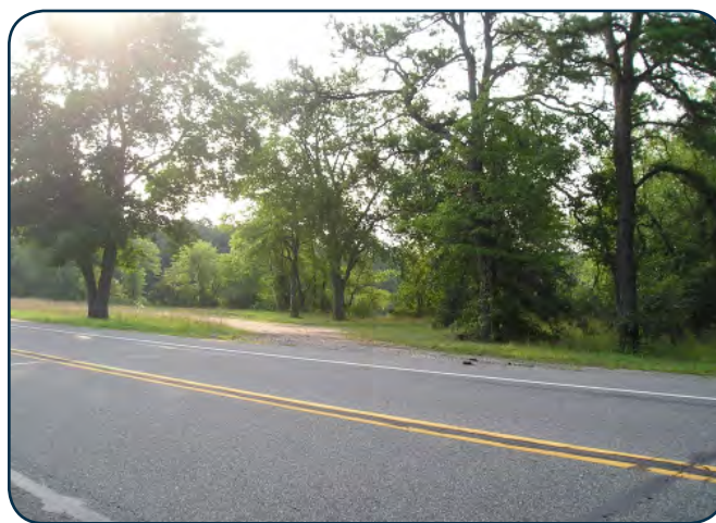
Rustic pull off area on the Rockefeller Memorial Highway (Route 70). (Courtesy of NJDOT.)
