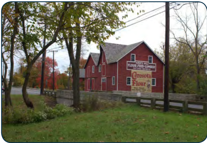
The early 20th-century concrete bridge at Kirby's Mill in Medford Township, Burlington County was replaced with a similar concrete bridge with eight feet additional width. The scoring on the new concrete parapets mimicked that of the historic bridge. Adjacent historic buildings were not disturbed. (Courtesy of the New Jersey Historic Preservation Office.)
