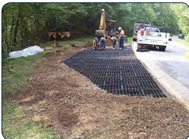
Construction of a stabilized grass pulloff area, with a geoblock base, along the Foothills Parkway in Great Smoky Mountains State Park, Tennessee, during (left) and after construction (right). (Courtesy of the Federal Highway Administration.)
