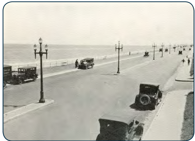
Ocean Drive, Long Branch, Ocean County. (Courtesy of NJDOT.) Note the curbed median, sidewalk, and period light fixtures.
