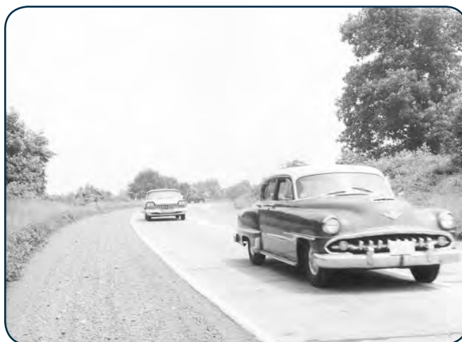
Note the gravel shoulders along Route 31, Hunterdon County, 1959. (Courtesy of NJDOT.)
