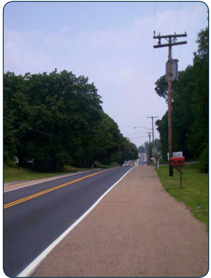
TyreGrip applied to the paved shoulder creates a safe surface for cyclists and drivers, and maintains the two-lane rural character of the road. (Courtesy of NJDOT).
