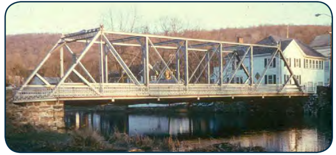
The Pratt through truss structure of the Califon Bridge is evident in this pre-rehabilitation photo. (Courtesy of NJHPO).
