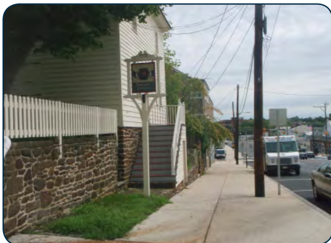
The new concrete curb was tinted to match the historic bluestone curb on a bridge over the Cohansey River in Bridgeton, Cumberland County. (Courtesy of NJDOT.)
