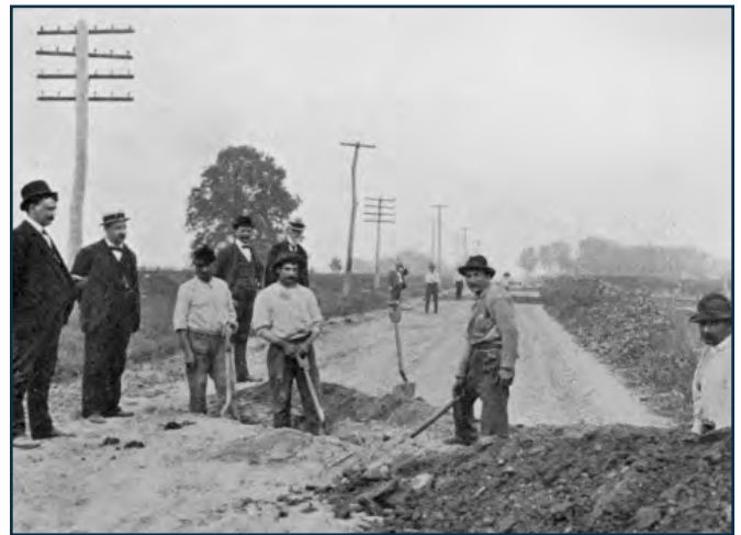
Installing under-draining system under Old York Road, Mercer County, date unknown.
