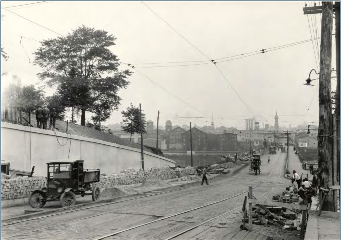
Construction to widen the Raritan River bridge between New Brunswick and Highland Park, Middlesex County, date unknown. (Courtesy of the University of Michigan, Transportation History Collection, Special Collections Library, Lincoln Highway Digital Image Collection.)
