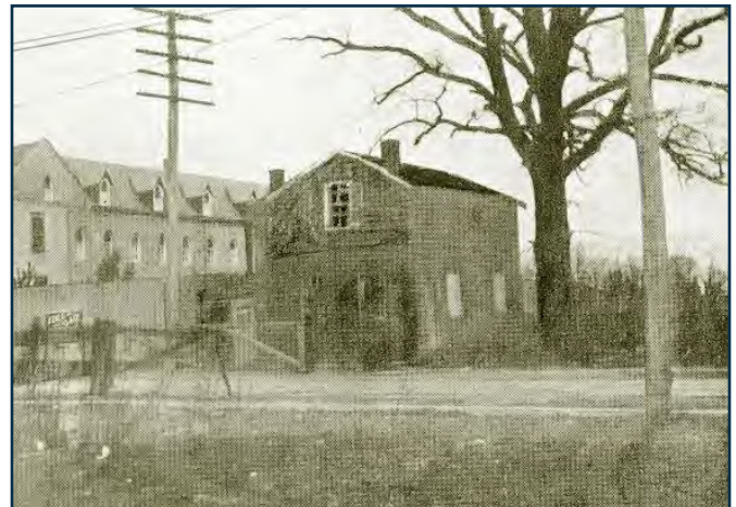
Toll gate and toll house on Haddon Avenue below Euclid Avenue on the Haddonfield and Camden Turnpike, Camden, date unknown.
