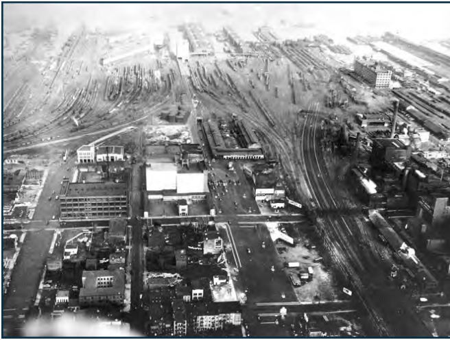
New Jersey Terminus of the Holland Tunnel, looking east, showing the exit and entrance portals and plazas, Jersey City, 1947.
