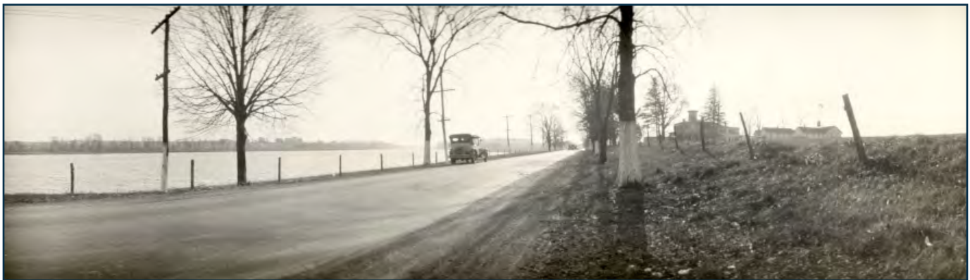
Looking west from the east end of Carnegie Lake near Princeton, New Jersey, 1923. (Courtesy of the University of Michigan, Transportation History Collection, Special Collections Library, Lincoln Highway Digital Image Collection.)
