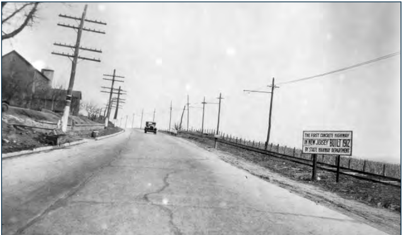
The first concrete highway, near New Village, Warren County, date unknown.
