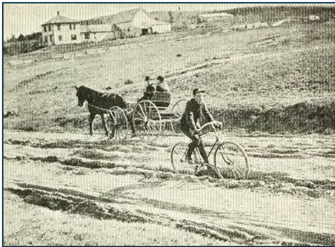
Rutting typical of undrained roadways, date unknown.
