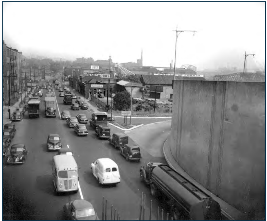
Route 21 (McCarter Highway), Newark, Essex County, 1950.
