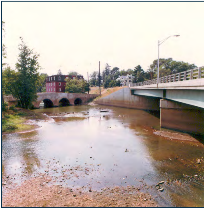
Stone bridge over the Millstone River in Kingston, built in 1798, adjacent to its 1970 replacement carrying Route 27.
