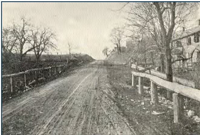
Morris Turnpike, Lopatcong Township, Warren County, after improvements, date unknown.
