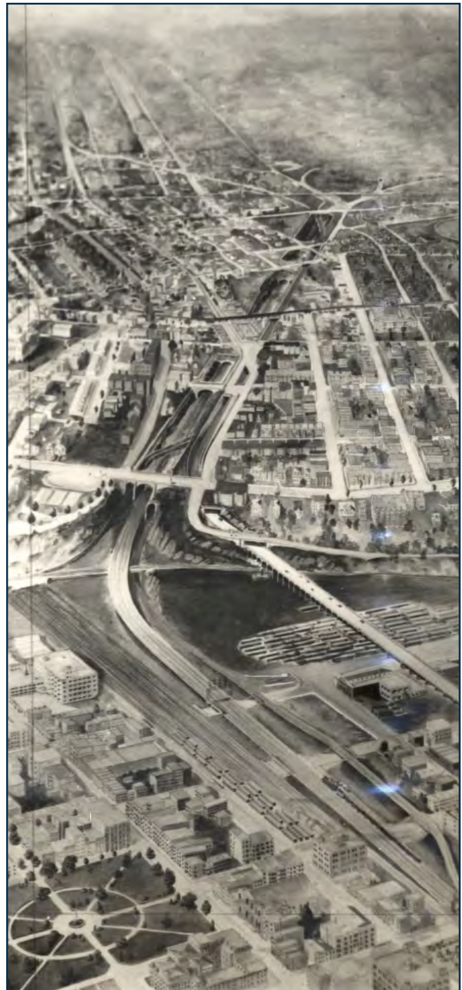
Rendering of the proposed Lincoln Highway at the emergence of the highway tunnel in Jersey City, date unknown. Note the proximity and concentration of rail and automobile traffic at this new link to New York City. (Courtesy of the University of Michigan, Transportation History Collection, Special Collections Library, Lincoln Highway Digital Image Collection.)
