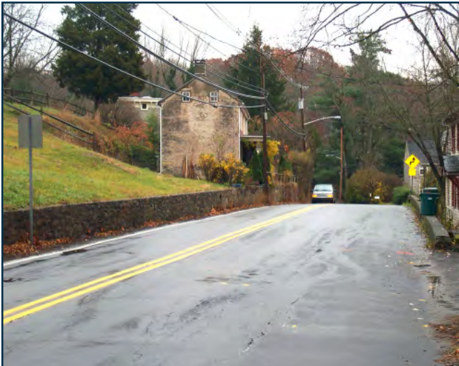
Delaware River Drive (Route 29), Stockton, Hunterdon County, 2000.
