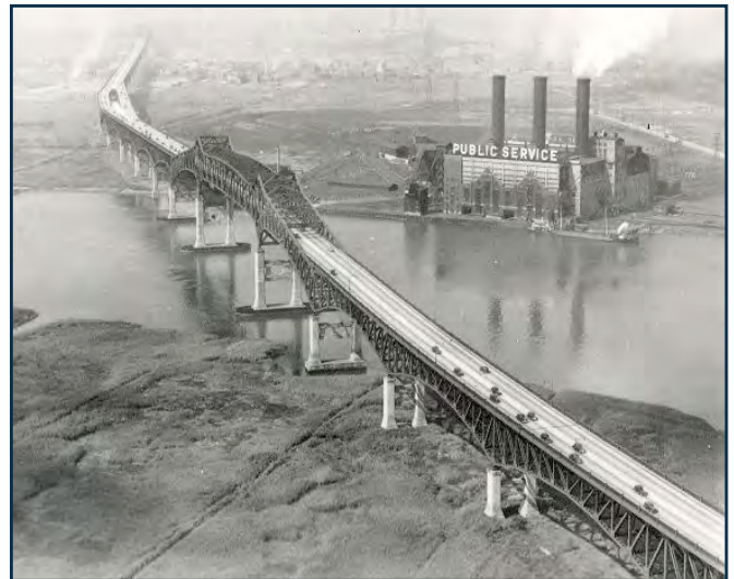
Route 1 & 9, Pulaski Skyway, between Newark and Jersey City, Essex and Hudson counties, date unknown.
