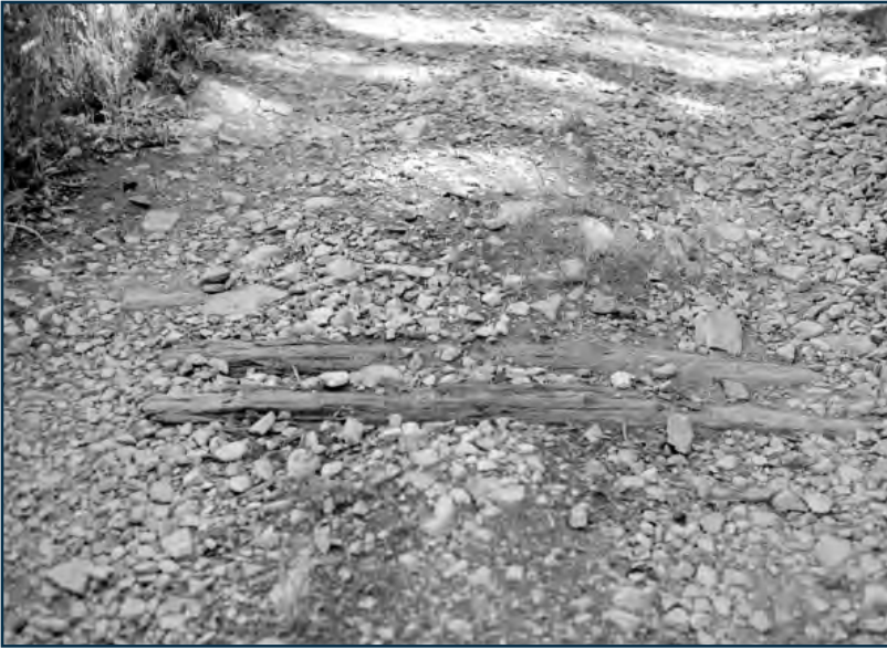
A section of corduroy road logs remaining on Genoa Peak Road in Nevada. (HAER NEV.3-SPU.V.1B-13. National Park Service. Photography by Larry Kingsbury, 1995.)
