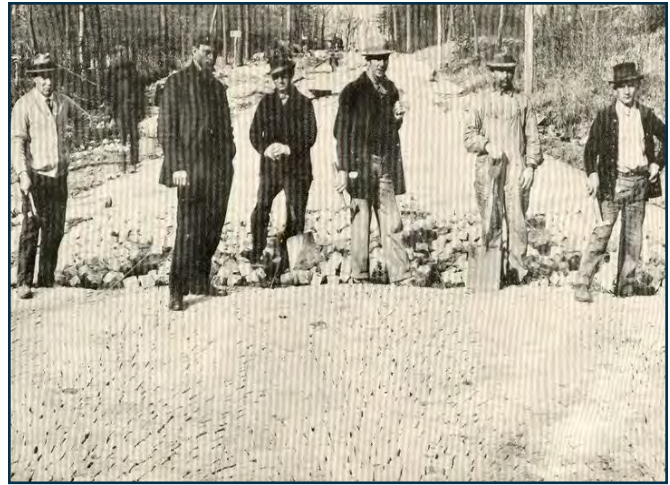
Installation of Durax Pavement on Morris Avenue, Essex County, date unknown. Durax consisted of granite blocks laid over a concrete foundation with a sand-cement paving bed and cement or mastic filler between the blocks.
