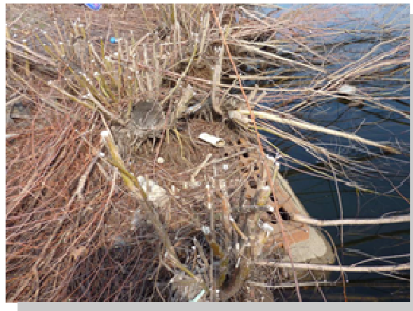
Overgrown vegetation interfering with wet pond outlet
