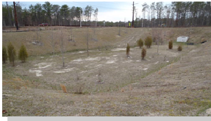
One of the stormwater basins evaluated
