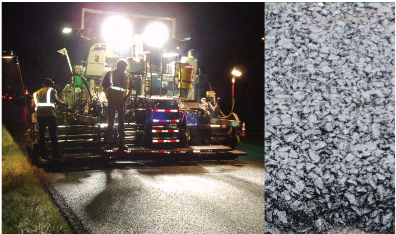
I-95 Rubberized "Quiet" Roadway Asphalt
