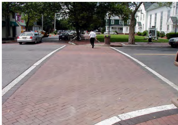
Rt. 88 crosswalk in historic Lake- wood
