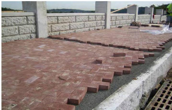
Rt. 18 New Brunswick brick sidewalk under construction
