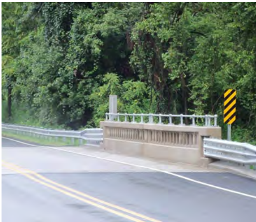
Jacksonville-Jobstown Road, Burlington County example of punched-out parapet in vicinity of Jacksonville Historic District (future application on Rt. 9 in West-cunk Historic District)
