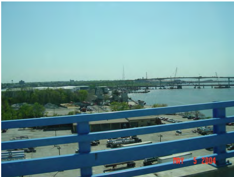
Rt. 9 Edison bridge over the Raritan River
