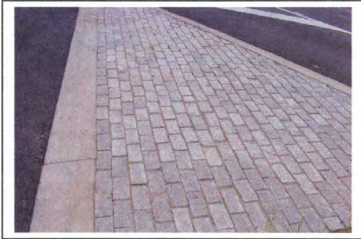
Granite pavers on median used as crossing refuge and to separate traffic
