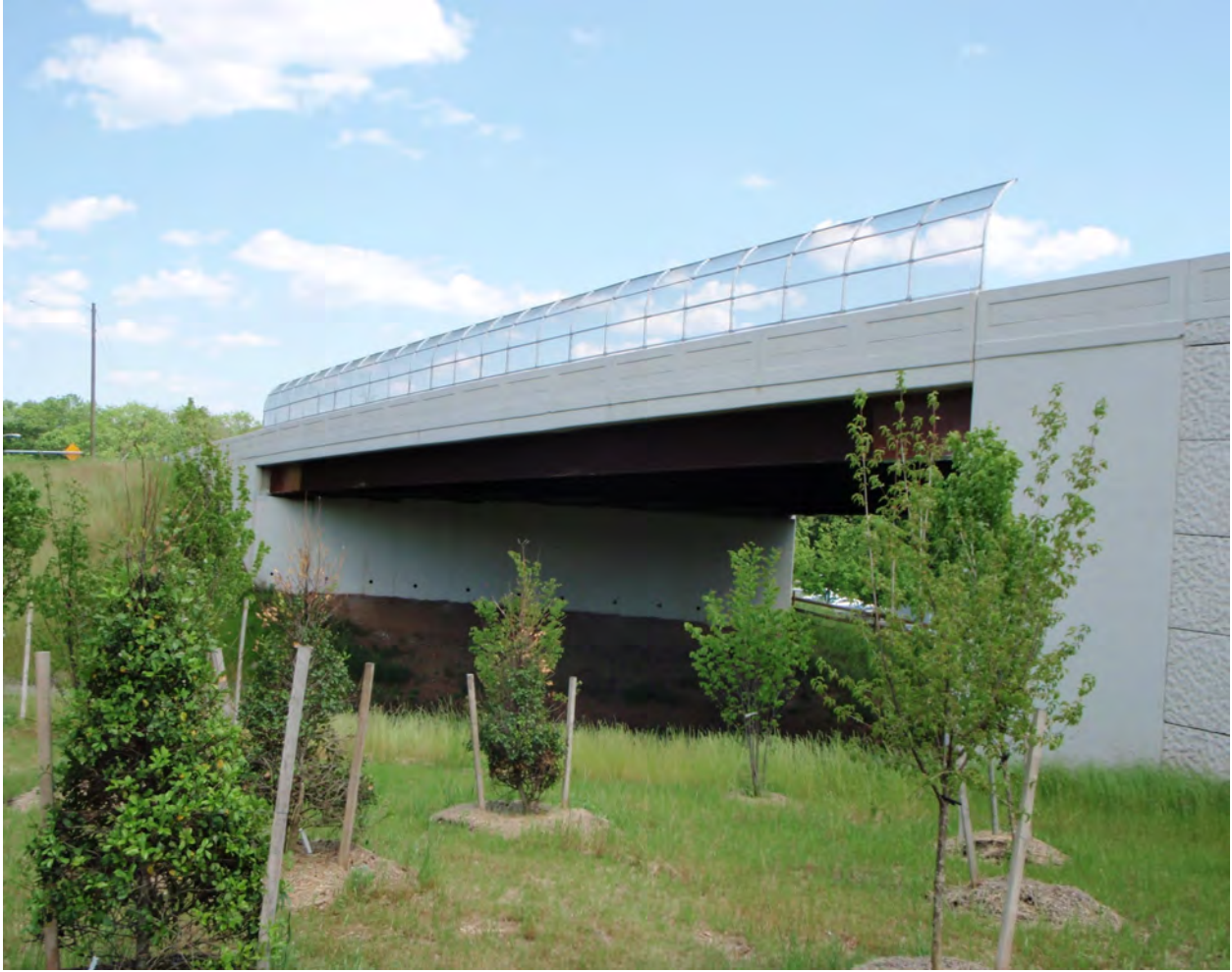
Amwell Road bridge over the historic railroad
