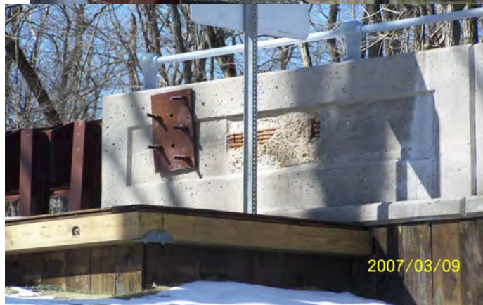
Interpretative sign is located above embedded sample of historic Lutens technology of original bridge
