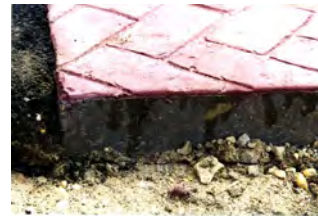
Rt. 30/130 Collingswood Circle showing tinted and stamped concrete to evoke laid brick (profile below)
