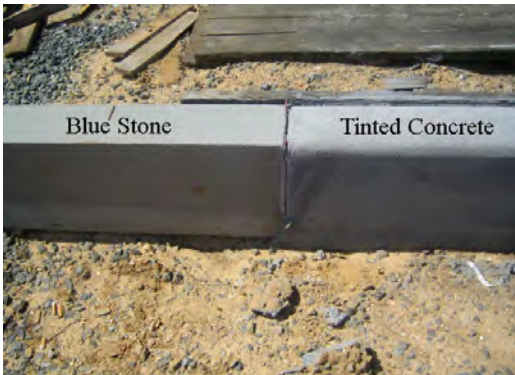
Rt. 49 Cohansey River in Bridgeton Historic District tinted concrete to match existing blue stone curbing
