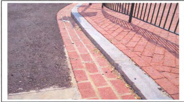
Rt. 29 Deck Park granite curb with brick gutter in Lambertton Historic District
