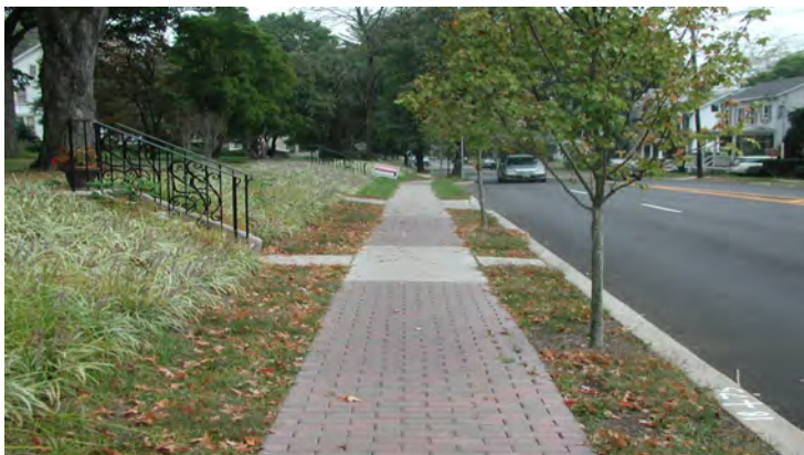
Rt. 173 sidewalk in Clinton Historic District using brick pavers and concrete
