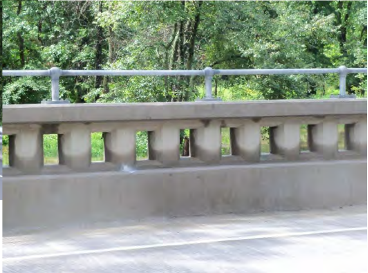
Jacksonville-Jobstown Road, Burlington County example of punched-out parapet in vicinity of Jacksonville Historic District (future application on Rt. 9 in West-cunk Historic District)
