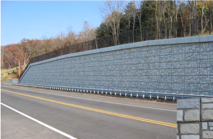
Rt. 31 Readington Township, Rowland's Mills Historic District
