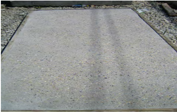
Rt. 49 over Cohansey River exposed aggregate sidewalks to evoke 1920s highway era within the Bridgeton Historic District
