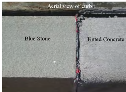
Rt. 49 Cohansey River in Bridgeton Historic District tinted concrete to match existing blue stone curbing
