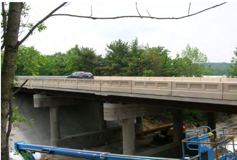
Jacksonville-Jobstown Road, Burlington County example of punched-out parapet in vicinity of Jacksonville Historic District (future application on Rt. 9 in West-cunk Historic District)
