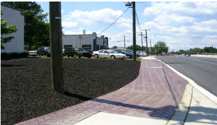
Rt. 30/130 Collingswood Circle showing tinted and stamped concrete to evoke laid brick (profile below)
