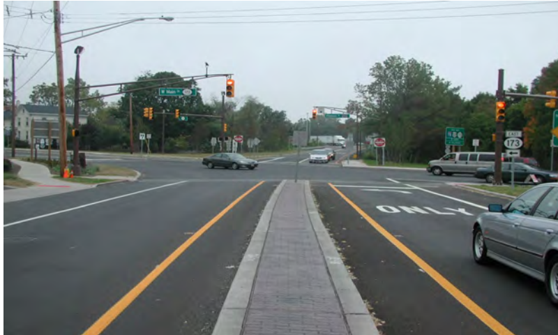
Rt. 173 in Clinton Historic District with stamped concrete to evoke granite pavers. It is mountable by turning emergency vehicles; stamping will not dislodge
