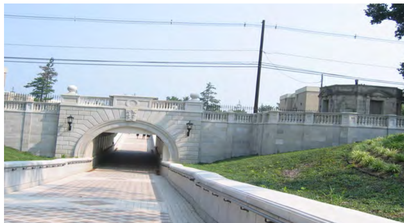
Rt. 71 tunnel at Monmouth University allows students easy access under highway
