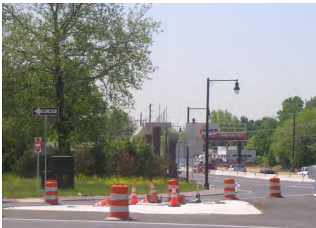
Rt. 30/130 Collingswood Circle
