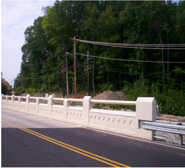
Hope Road over historic rail- road district, Blairstown vicinity, Warren County
