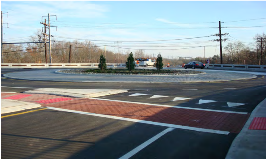
Crosswalk at roundabout at Alexander Road Bridge over Northeast Corridor Railroad Historic District, West Windsor
