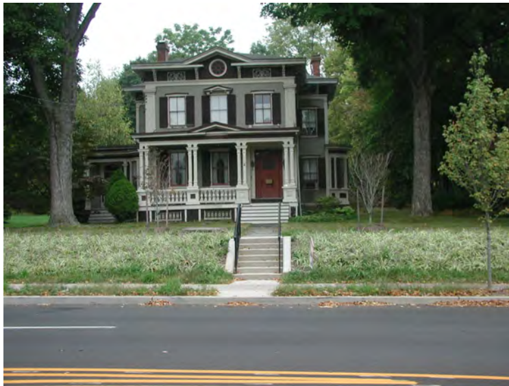
Rt. 173 Clinton Historic District received new retaining walls, plantings, and gateway treatment
