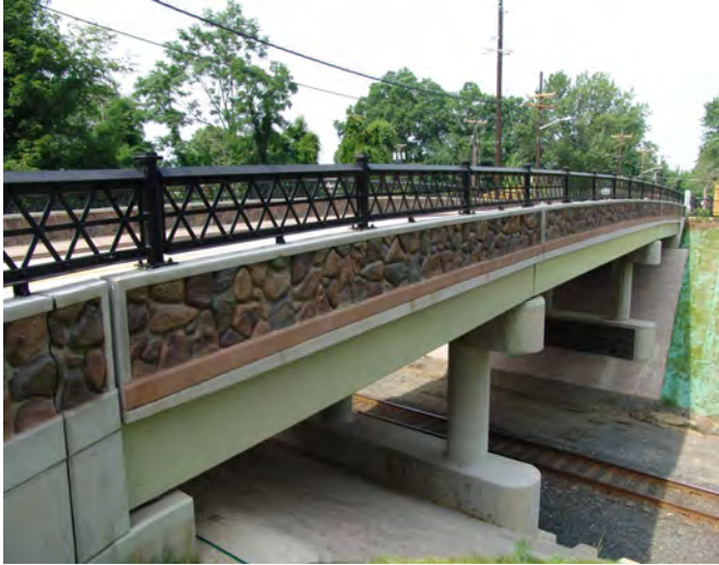
Maple Avenue in Haddon Township over Camden and Atlantic Railroad Historic District
