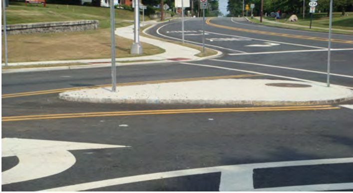
Rt. 124 and Kings Road, near Drew University, sidewalk and island after intersection improvements near Old Main Delaware, Lackawanna and Western Railroad Historic District and the Ridgedale Avenue Foot Bridge in James Park
