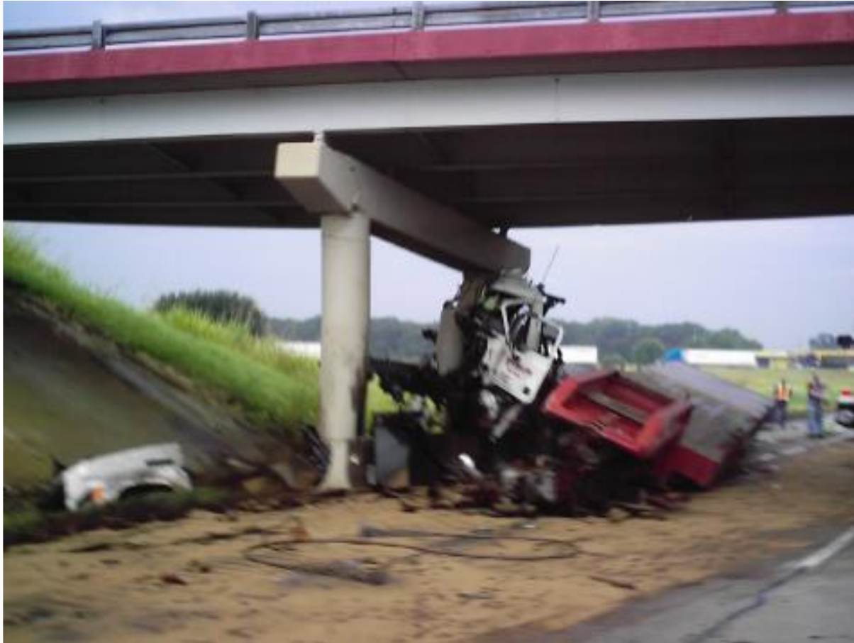
Truck impact on Mile Post 519 Bridge over IH-20, Canton, TX
