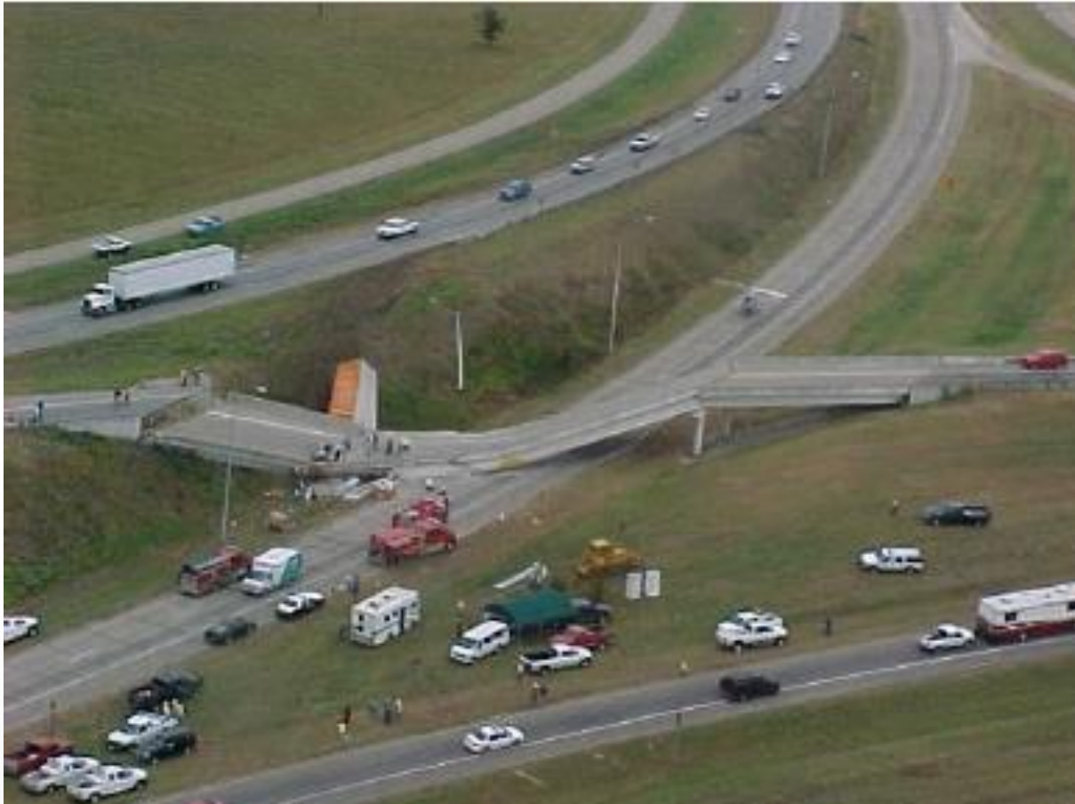
Truck impact on SH-14 Bridge Over IH-45, Corsicana, Texas
