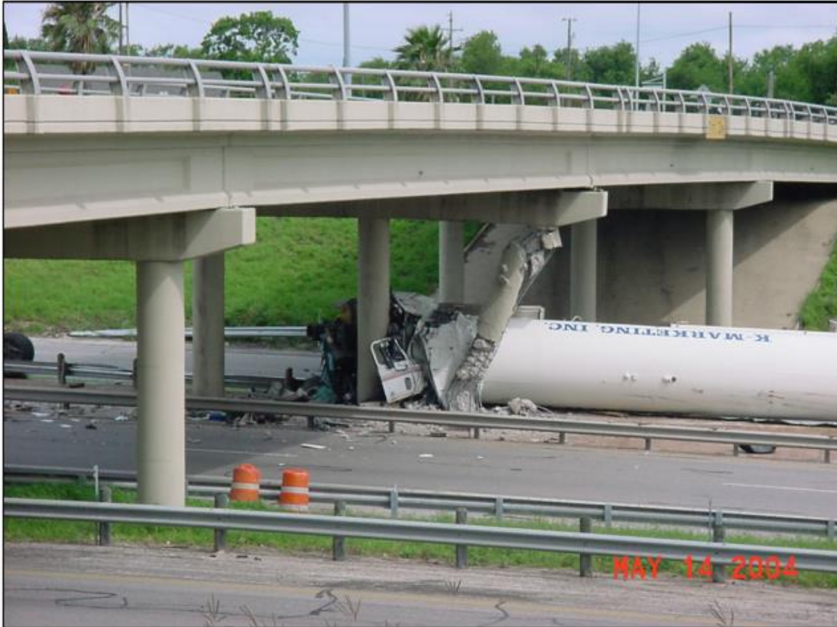
Truck Impact on Piers of Tanchua Street Bridge over IH-37, Corpus Christi, Texas on May 14, 2014.
