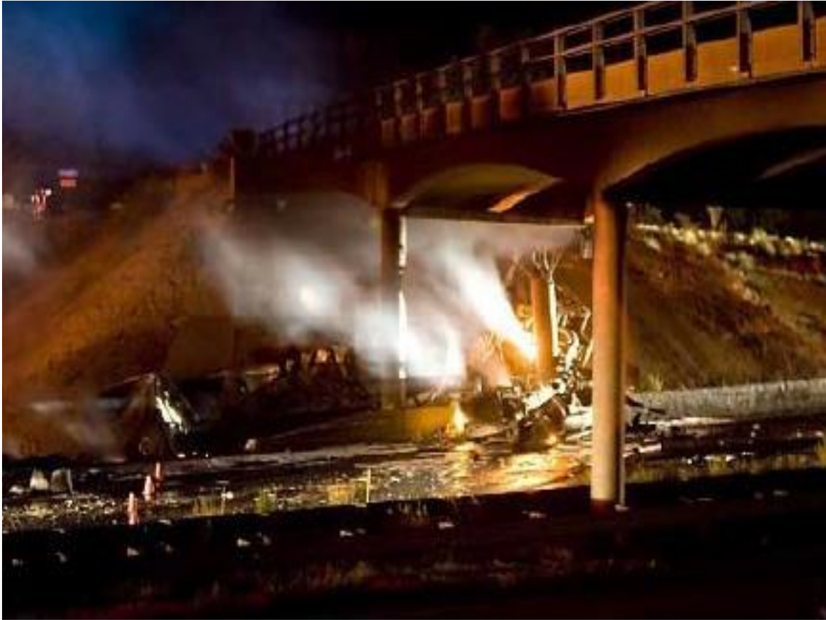
Truck impact on Bridge on 26 ½ Road over IH-70, Grand Junction, Colorado
