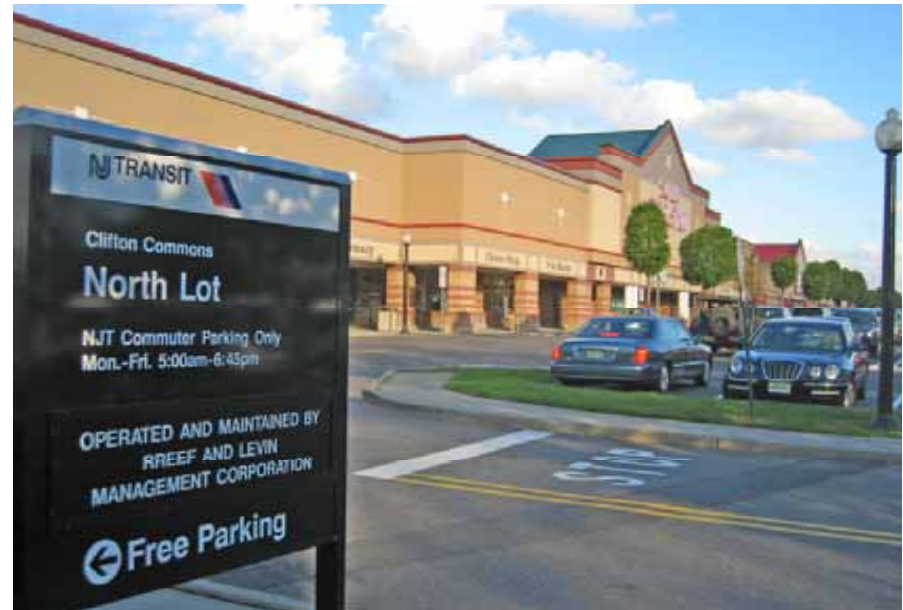
Shared parking at a Clifton shopping center accommodates transit users on weekdays.
