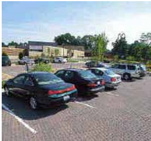
Permeable interlocking pavers and biofiltration swales can reduce environmental impacts. Source: Sikich and Kelsey (left), Wendi Goldsmith (right).
