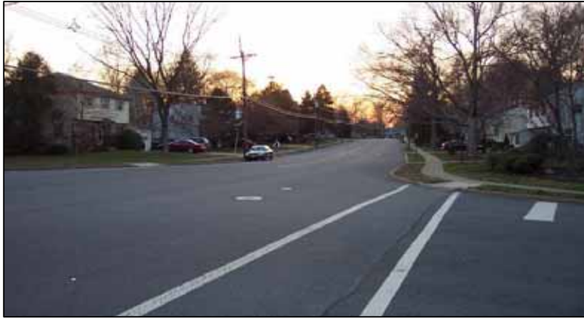
This overly wide residential street encourages speeds far above the 25 mph limit.
