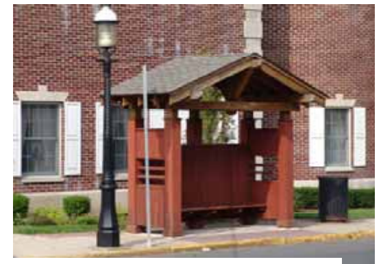
This bus shelter in Metuchen is simple, yet elegant, with a light, airy open design, side openings so seated patrons can watch for the bus, a curbside tactile strip to help prevent falls, adjacent lighting and a trash receptacle.
