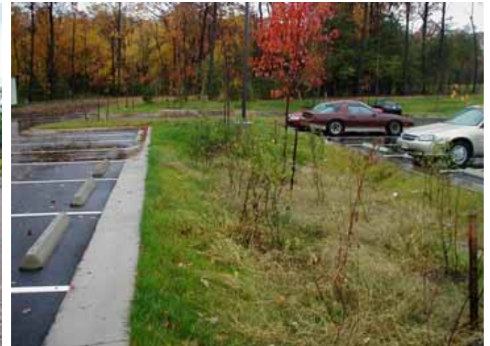
Permeable interlocking pavers and biofiltration swales can reduce environmental impacts. Source: Sikich and Kelsey (left), Wendi Goldsmith (right).
