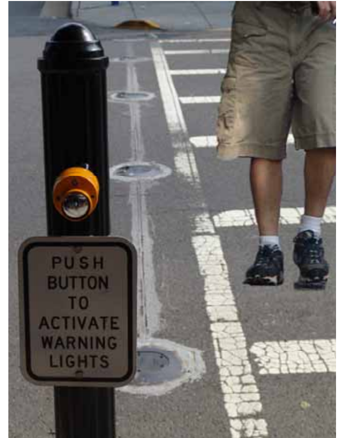
A lighted crosswalk in Metuchen.
