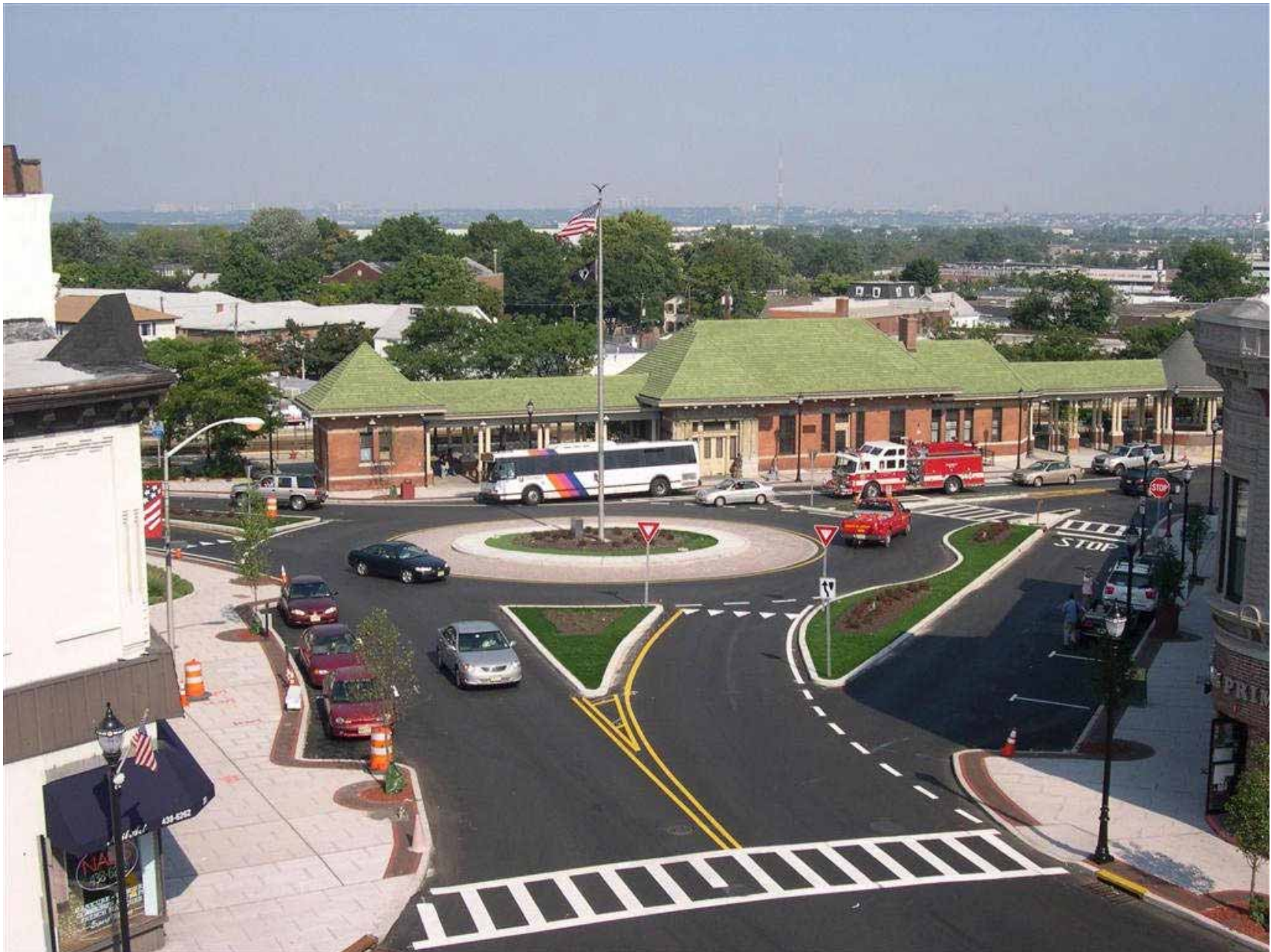
Roundabout in Rutherford slows and channels traffic.
