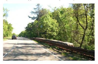
Existing photo of the metal guardrails in front of the original bridge rails on the New Jersey section of the Palisades Interstate Parkway
