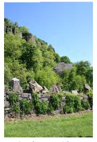
Invasive plant material attached to parapet wall
