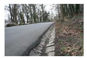
Existing photo of the stone gutter along Henry Hudson Drive. Note the raised asphalt surface.
