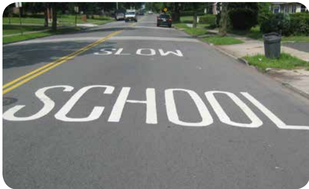
“Slow School” pavement markings on Glenwood Avenue in East Orange, NJ. Image: The RBA Group
