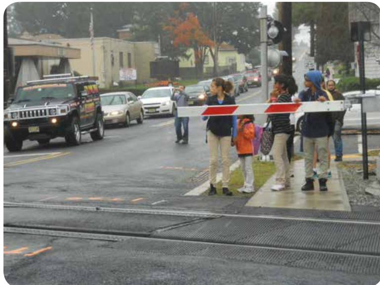
Students waiting behind a pedestrian gate to cross the tracks in Garfield, NJ. Image: The RBA Group
