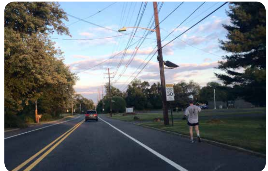
Burlington County has been striping 6-inch edge lines on shoulders along roadways with high bicyclist and pedestrian use, including this section of County Route 528 in a school zone in Bordentown Township. Image: NJDOT
