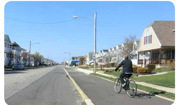
A raised cycle track in Ocean City, NJ. Image: The RBA Group
