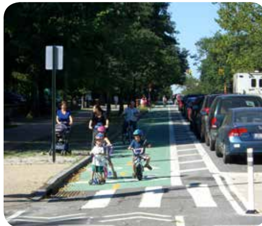
Two-way cycle track buffered by on-street parking. Image: NYC.gov
