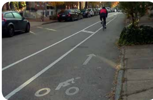
A buffered bike lane in Philadelphia, PA. Image: The RBA Group
