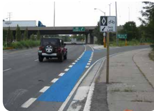
Providing bicycle facilities leading to and through the ramp improves visibility. Image: Cleanairpartnership.wordpress.org
