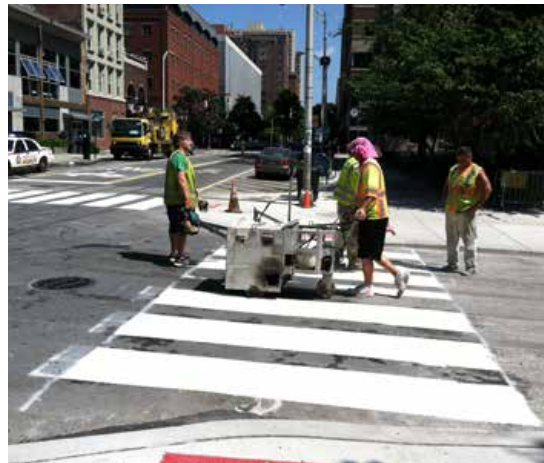
Installing high visibility crosswalks in Hoboken, NJ. Image: The RBA Group
