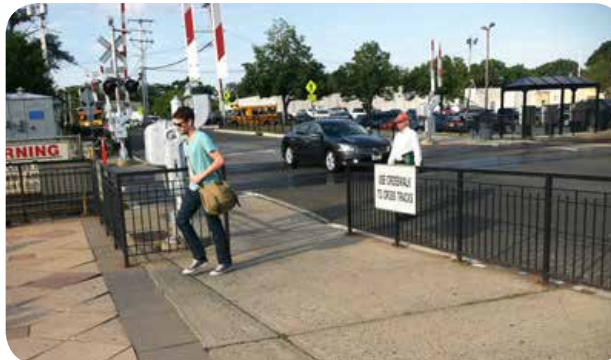
Fencing at NJ TRANSIT's Aberdeen-Matawan Station. Image: The RBA Group
