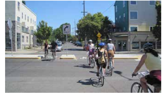
Example of a raised median along a bike boulevard. Image: NACTO
