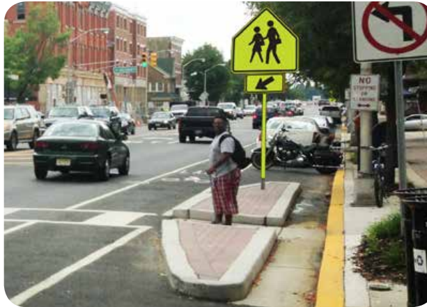
A mid-block storm-water curb extension example, Route 45 in Woodbury, NJ. Image: NJDOT
