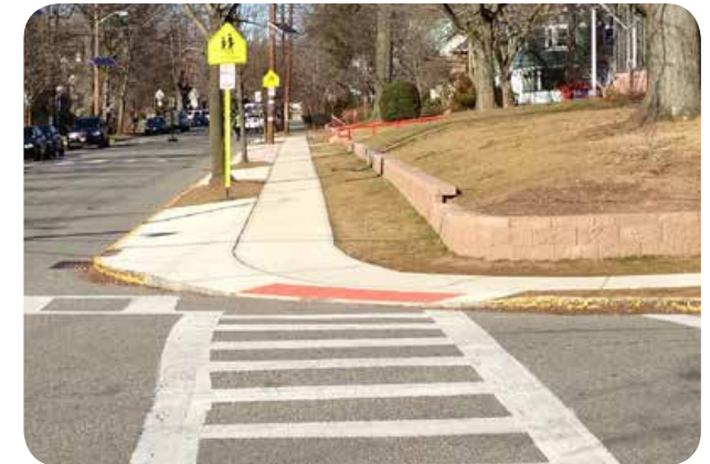
Diagonal curb ramps are not desirable because they force pedestrians into the intersection and are more difficult for visually-impaired people to determine the correct crossing location and travel direction. Image: Arterial
