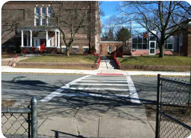
Fencing funnels pedestrians to the signed and well-marked midblock crosswalk in front of the Watchung School in Montclair, NJ. Image: The RBA Group
