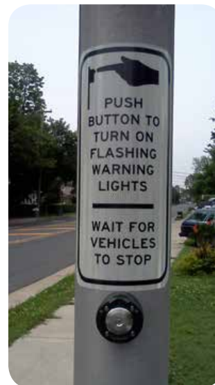
An RRFB signal has been installed in Atlantic County at the intersection of Old Tilton Road (NJ 687) and the Linwood Bikepath. Image: The RBA Group
