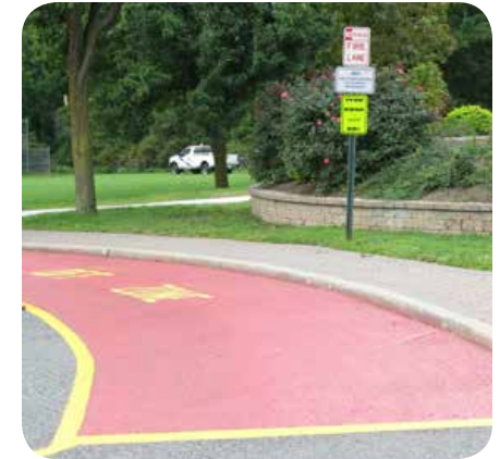
Motor Vehicle Drop-off Zone at the Orchard School in Ridgewood, NJ. Image: The RBA Group
