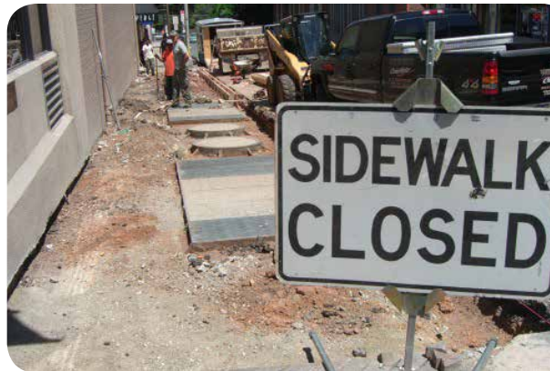
Sidewalk closed for repairs. Image: VTC
