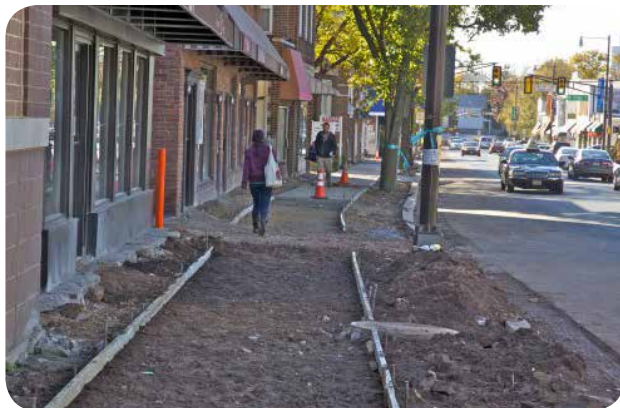
Sidewalk ready to be poured. Image: VTC
