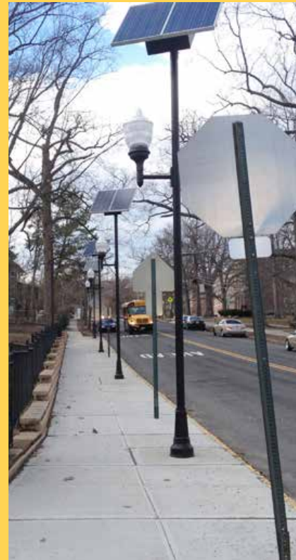
Newly installed solar powered lighting along North Fullerton Avenue. Image: Arterial
