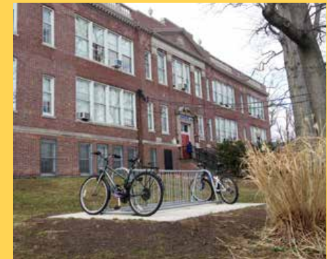
Newly installed concrete pad and bike rack at the front entrance of the school. Image: Arterial
