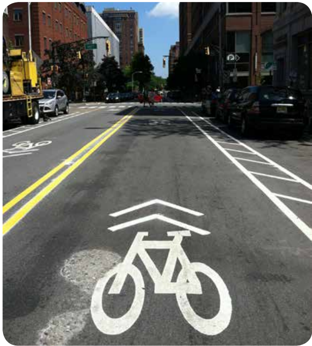
Newly-installed “sharrow” in Hoboken. Image: The RBA Group
