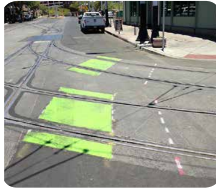
Green pavement markings in Tuscon, AZ indicate where cyclists may cross streetcar tracks at as close to perpendicular as possible. Image: bicycletuscon.com
