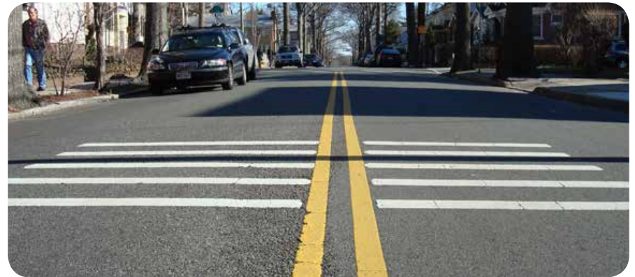
Rumble strips in Newark, NJ. Image: The RBA Group
