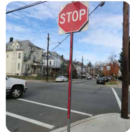
Reflective tape on stop sign post in Newark, NJ. Image: The RBA Group
