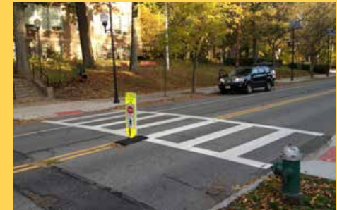
Newly painted high visibility, continental crosswalk and in-pavement “Stop for Pedestrian” crossing sign. Image: Arterial
