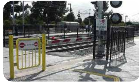
An emergency exit swing gate is used in conjunction with an automatic pedestrian gate. It is designated for use only as an escape route for a pedestrian that remains between the track and a lowered automatic pedestrian gate. Image: FHWA
