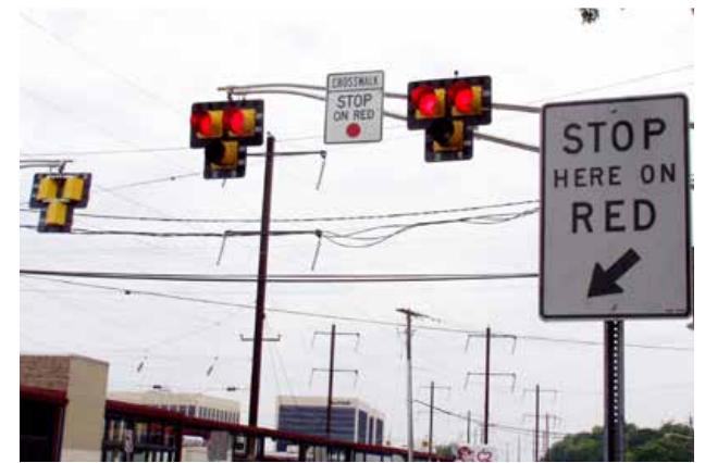
HAWK Signal across Route 27 to the Metropark Train Station. Image: NJDOT
