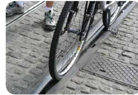
Bicycle tires can get stuck on the grooves between tracks. The safest way to cross rail tracks is as close as possible to a 90 degree angle. Image: BicycleGermany.com
