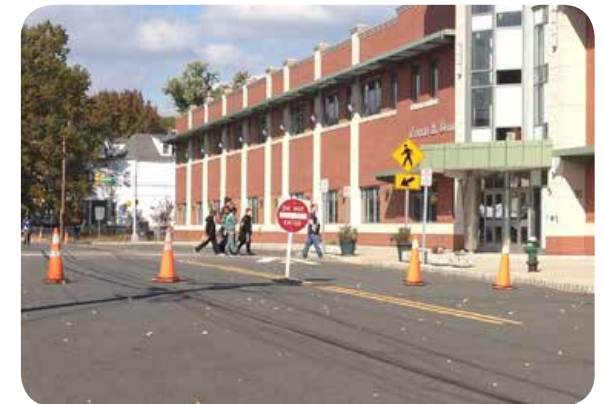
Temporary roadway closure in front of the Bullock School in Montclair, NJ. Image: The RBA Group
