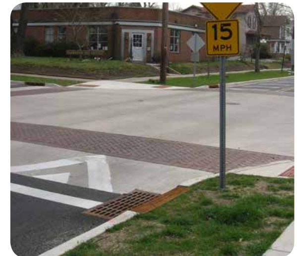
Raised intersection, Haddonfield, NJ. Image: VTC
