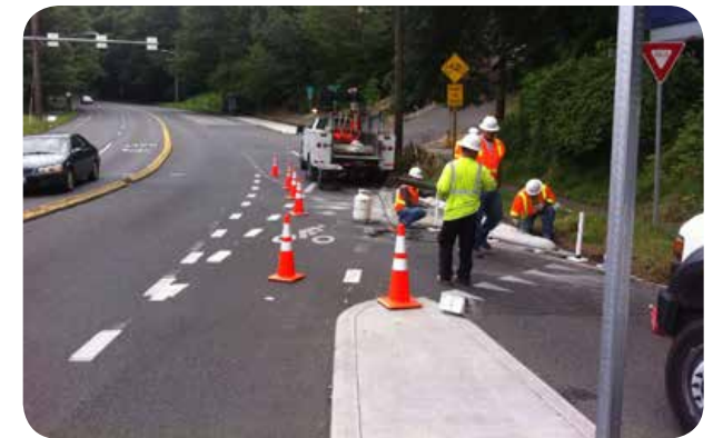
Seattle DOT installed a refuge median and curb extension at this right turn lane which narrows the travel way and forces motorists to slow down. Image: SeattleBikeBlog.com
