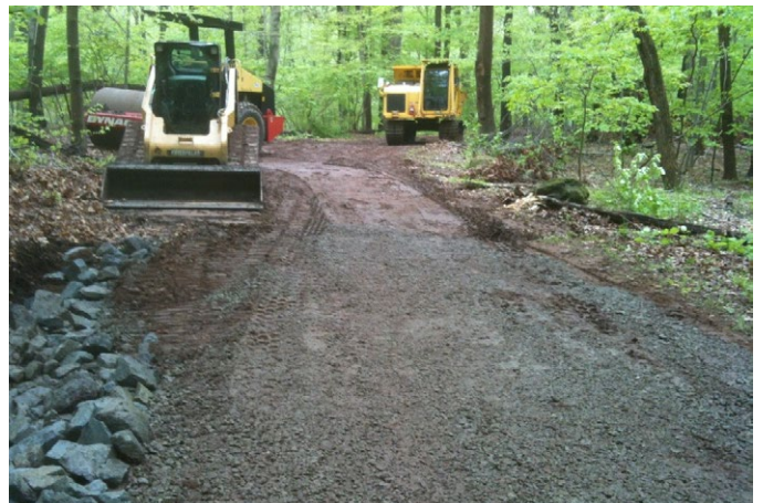
Trail construction at the South Mountain Reservation, Essex County
