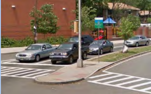
Pedestrian Refuge Area at the intersection of South Orange Avenue and Maybaum Avenue in Newark, NJ. Image: RBA
