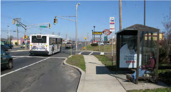
Access to the bus stop at Route 42 and Greentree Drive in Turnersville was improved with a bus pull out and sidewalks. Image: Parsons Brinckerhoff
