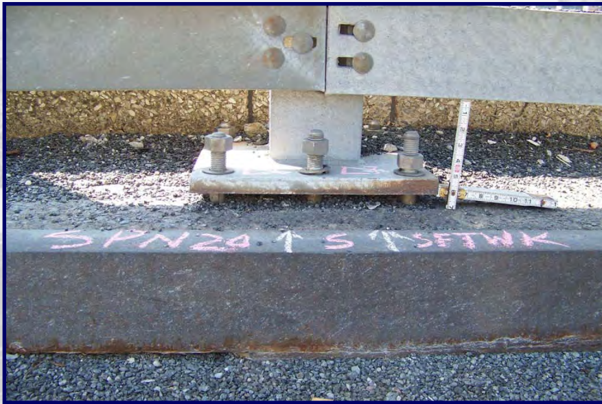
Span 20 (South bridge guiderail)
