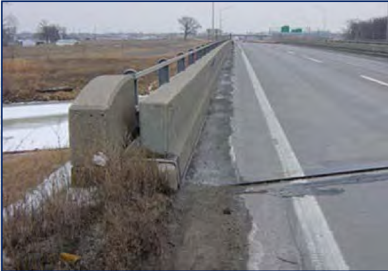
IOWA BARRIER CONCRETE BLOCK RETROFIT
