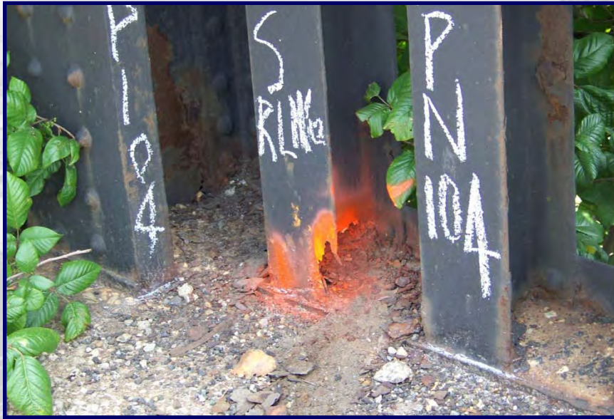
Span 104 south bridge railing near Pier 104 (Northbound Roadway)
