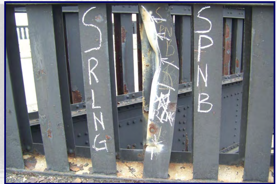
Span B South Railing (Newark Ramp)
