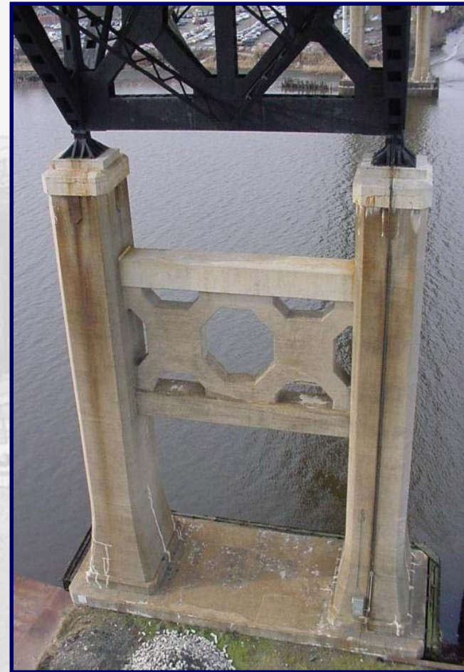
Reinforced Concrete Piers
