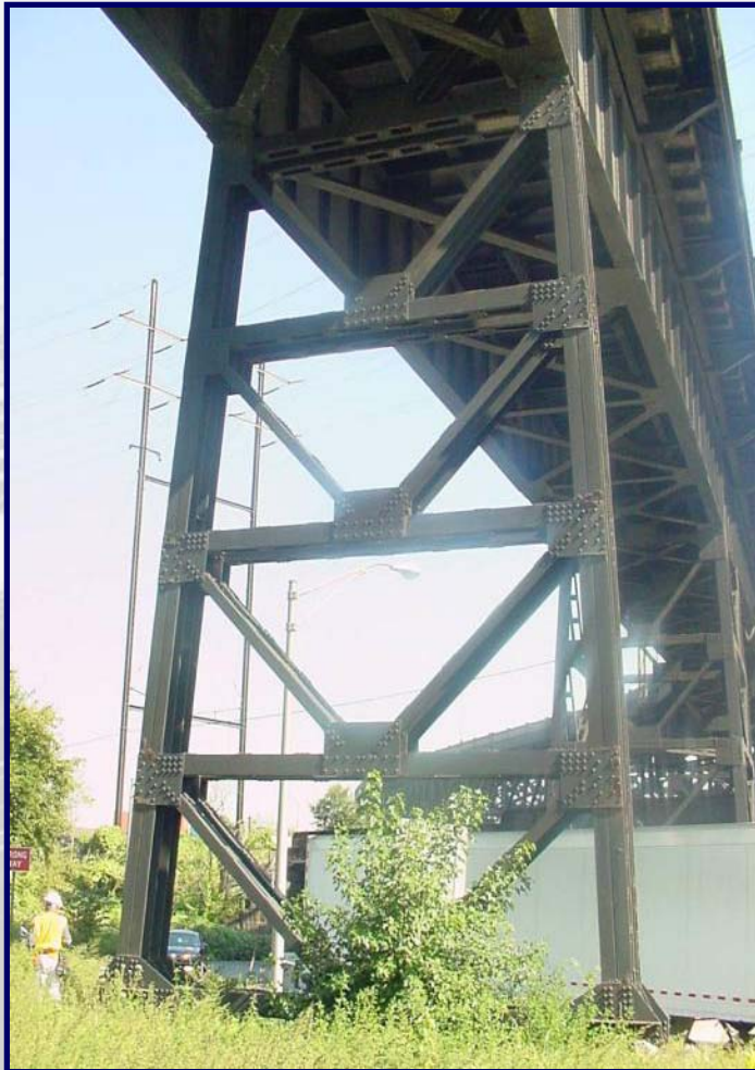
Steel Bent Pier
