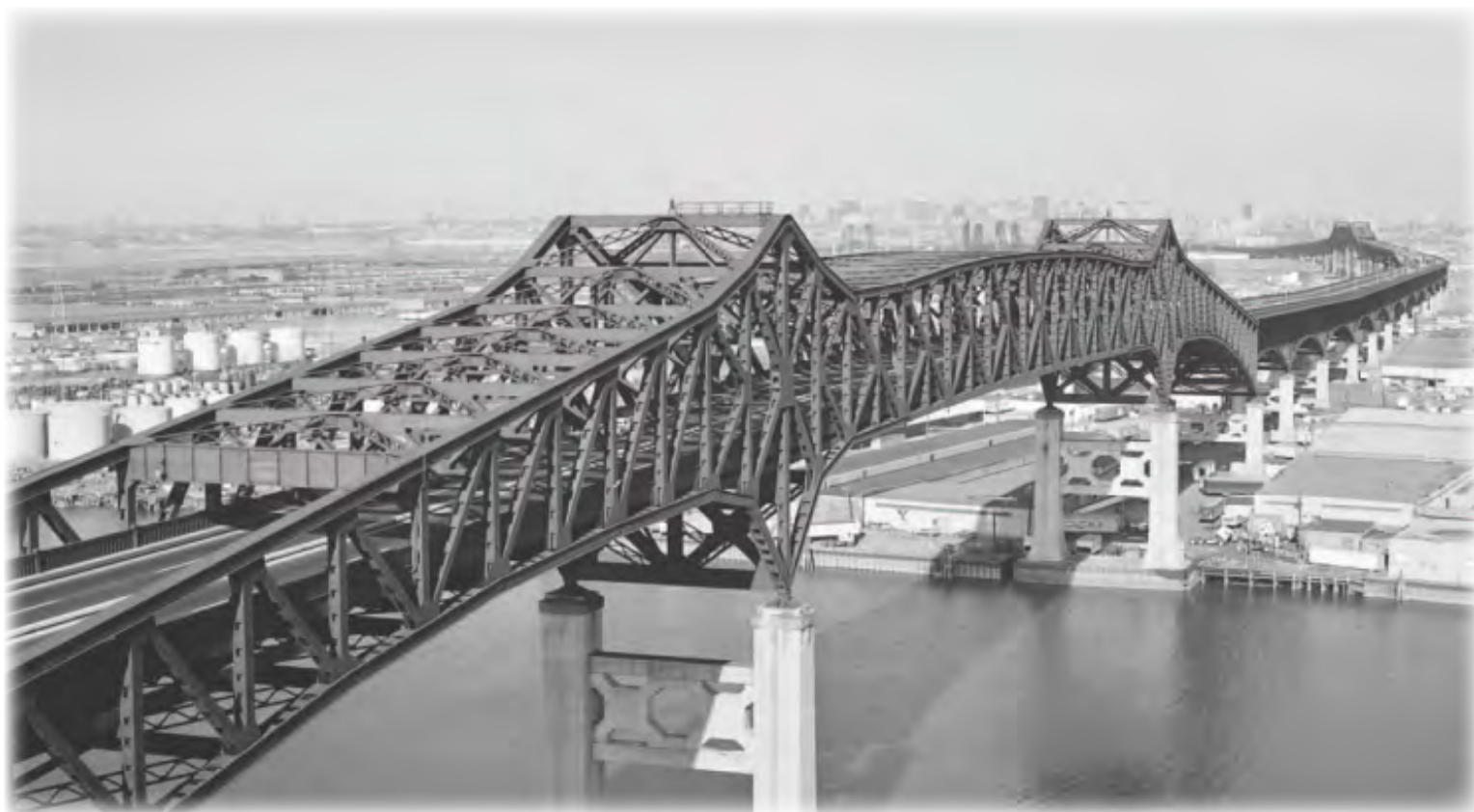
The Pulaski Skyway looking northeast over the Passaic River.
