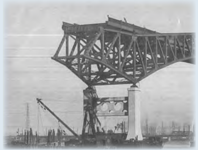
Pulaski Skyway during original construction
