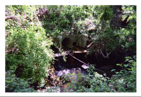
Photo Plate 39: View of inlet pipes conveying flow (Waters of the U.S. in Culvert) under Bellmawr Park. Note severe scouring of stream bank and structure.
