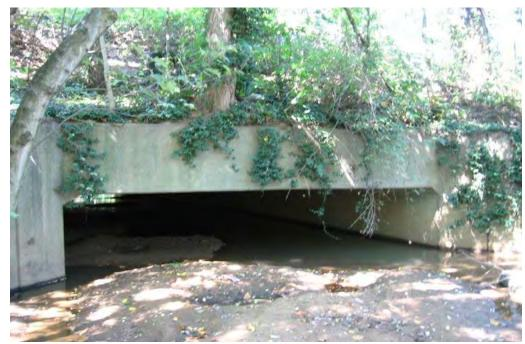
**Photograph 30**: Site 35, looking northwest at the eastern end of the Bell Road culvert. The channel of Little Timber Creek contains large deposits of sand and silt which restrict its flow. Removal of the deposits would reduce flooding.
