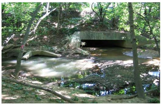
**Photograph 31**: Site 35, looking southeast at the western side of the Bell Road culvert, showing the silt and sand filled channel of Little Timber Creek. Removal of these silt deposits, snags and debris would allow the Creek to flow more freely, reducing flooding conditions. Adjacent wetlands also could be enhanced.
