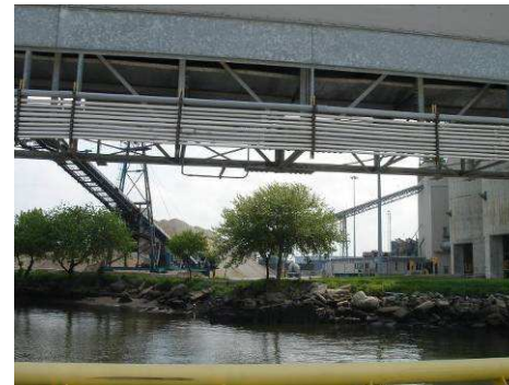
Environmentally Sensitive Concrete Operation at the Port
