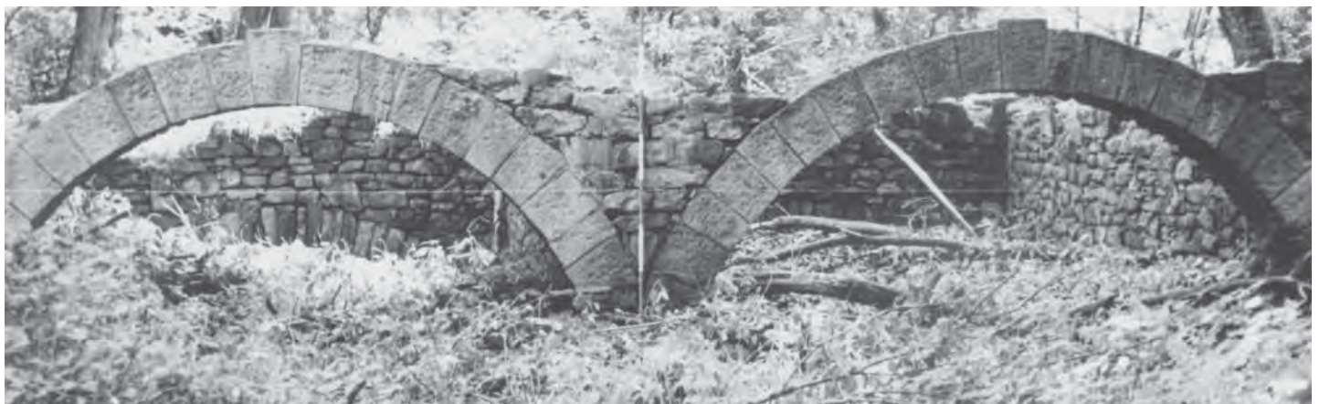
In the early 1990s substantial remains of the gristmill at Rowland's Mills still survived in the floodplain. This view shows the mill foundations with its arched raceway openings giving access to the wheel pit [Source: Louis Berger and Associates, Inc.].
