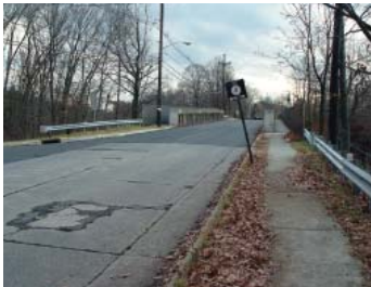
Highways require continuous maintenance to keep traffic flowing.
