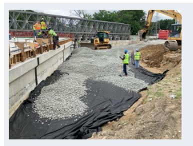
NJDOT has completed projects using ultra-lightweight foamed glass aggregate, a material made from 99 percent crushed container glass that can be used as fill under roadways and bridge approaches. Carbon emissions are reduced by using recycled products and reducing the amount of truck trips required to transport the lightweight material.
