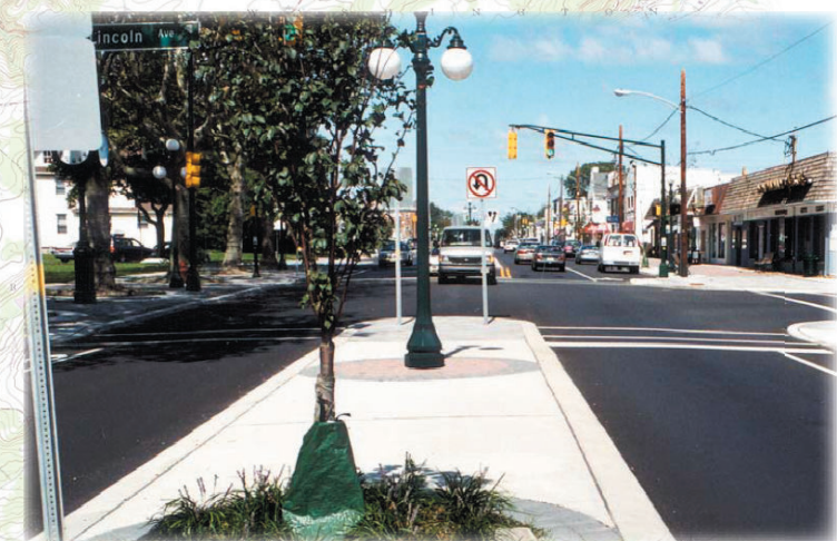
An NJDOT intersection improvement with traffic calming and pedestrian enhancements in Avon-by-the-Sea, Monmouth County, NJ.
